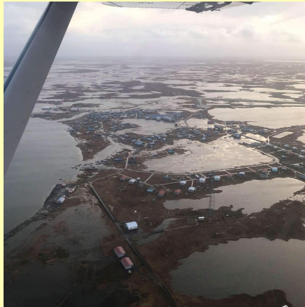
Figure 13. Photographic evidence of the flood event on October 4, 2018, in Kipnuk, Alaska.
