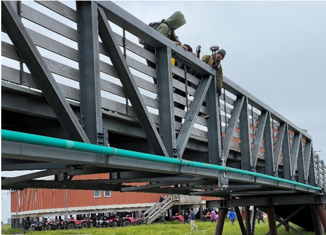
Figure 2. Stilltek iGage radar water level sensor installation in Kipnuk, Alaska, located on the south side of bridge.
