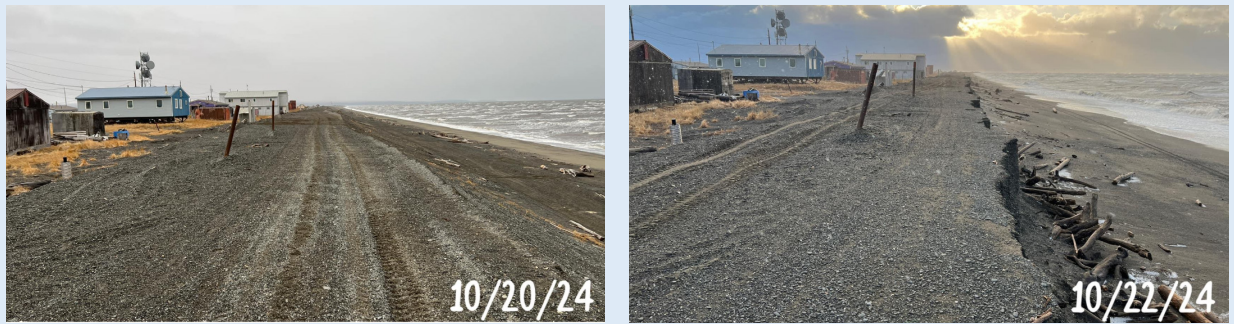
Figure 7. Before and after photographs of the berm in Shaktoolik, Alaska during the October 2024 flood event (credit: Gloria Andrew).
