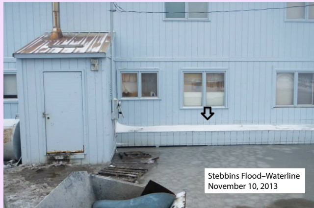
Figure 3. High water mark associated with the November 2013 flood event identified on the back exterior wall of the teacher housing building in Stebbins, Alaska.
