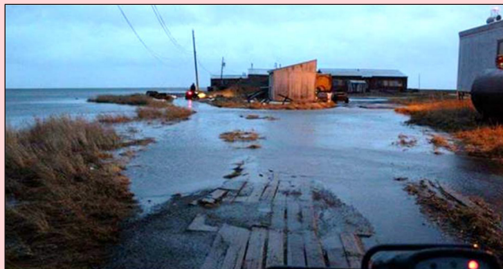
Figure 2. Flooding on access road to Head Start building on October 5, 2017, in Chefnak, Alaska (PDN, 2018).
