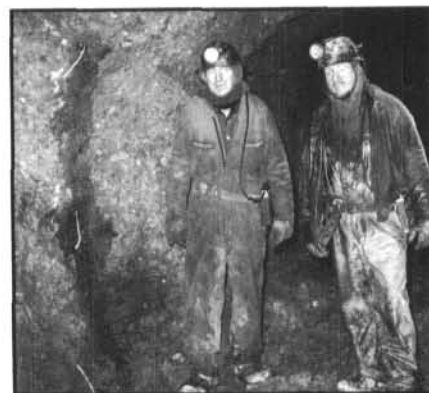
Figure 33. In the early days of Fairbanks, many placer operations were underground drift mines. Goldbearing gravels were hauled to the surface all winter and then washed in the summer when water was available. Technology now enables miners to excavate old stream channels 100 to 140 ft below the surface. At the Dome Creek Drift Mine, father and son operators prepare to blast gravel at the work face. (Photo by Bruce Campbell)
