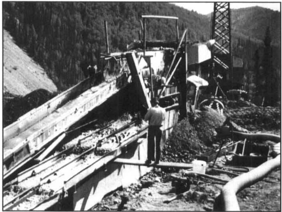
Figure 36. During the 1990 production season, Alaska's placer mines produced an average of 892 oz of gold. This typical operation uses a dragline to collect the gravel which goes through the washing plant. Once production is completed, the dragline will be used to recontour the mine site and reclaim the area. (Photo by Bruce Campbell)
