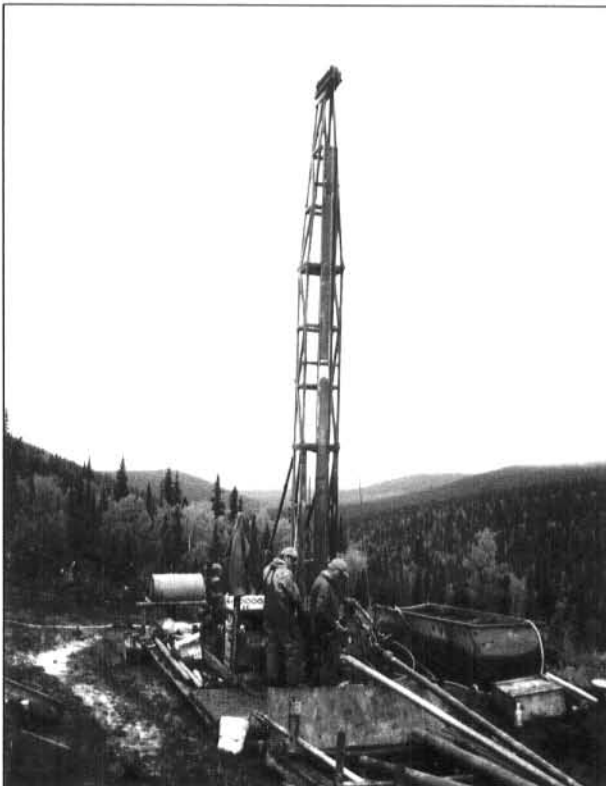
Figure 14. Ken Elordi and Bill Lowry of Boyles Brothers Inc. drill a test-water well in the Mystery claim area of the Nixon Fork project. Aquifer studies were initiated by Nixon Fork Mining Co., operator of the project during the 1993 development program. (Photo by Richard Flanders)
