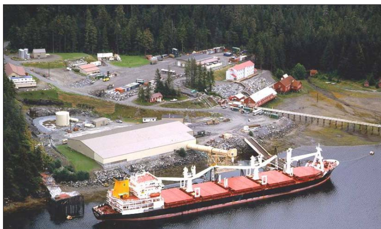
Figure 33. The ore concentrate loading marine terminal at Greens Creek Mine on Admiralty Island. Concentrates are trucked 9 miles from the mine site to the terminal. The Hawk Inlet camp is shown behind the loading facilities. Photo courtesy of Greens Creek Mining Co.
