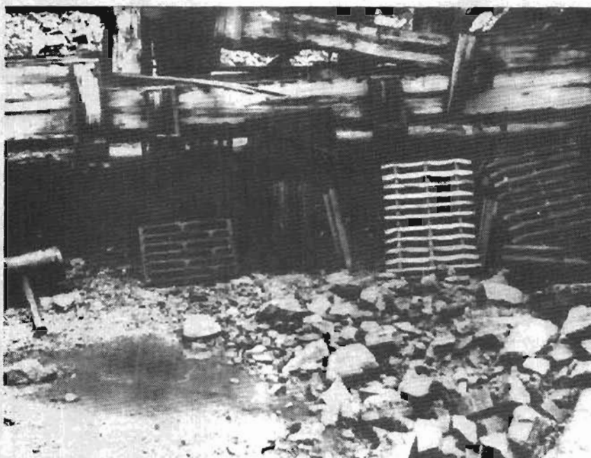
Fig. 12 - Variety of riffles used by Heine Carstens on Portage Creek
