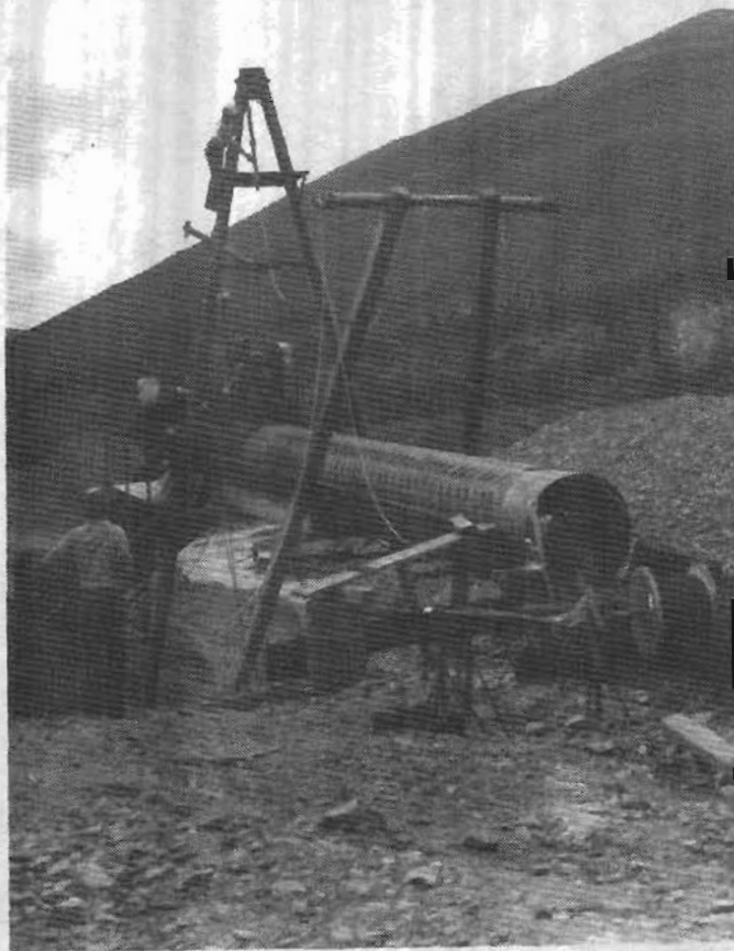
Suspended trommel screen and sluice combination.
