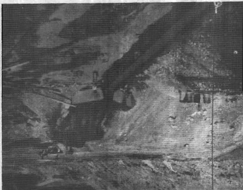
Fig. 3 - Pushing Gravel to a sluice plate at Olive Creek Mines
