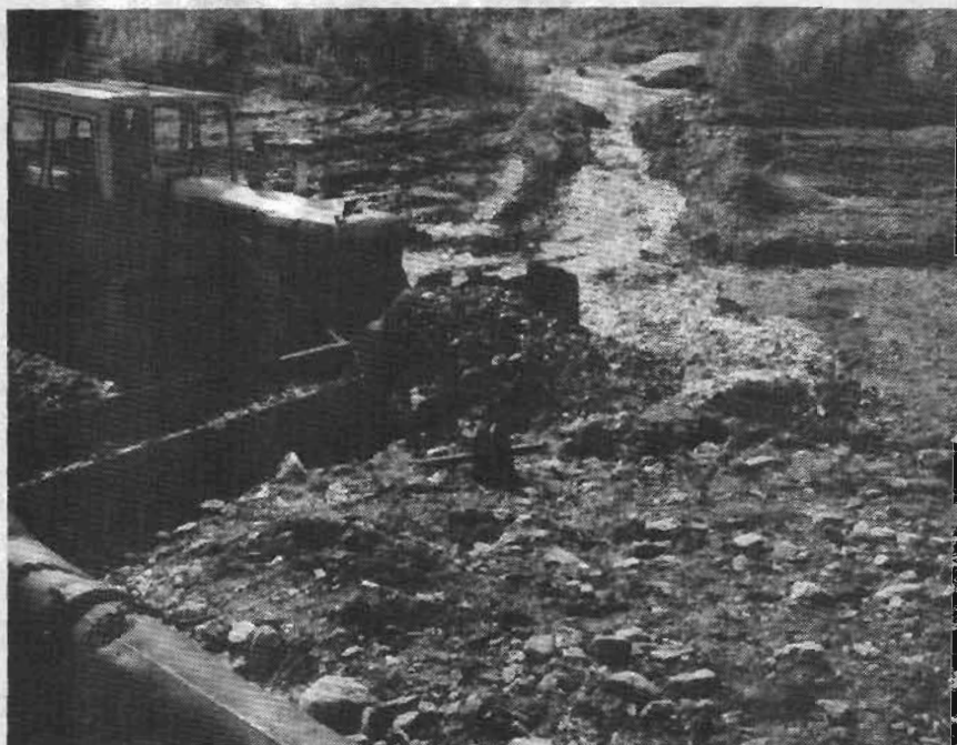
Tailings disposal below conventional sluice box.
