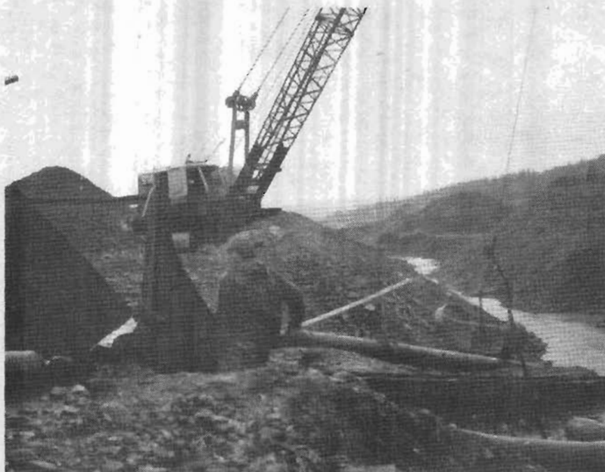
Dragline setup for tailings disposal.
