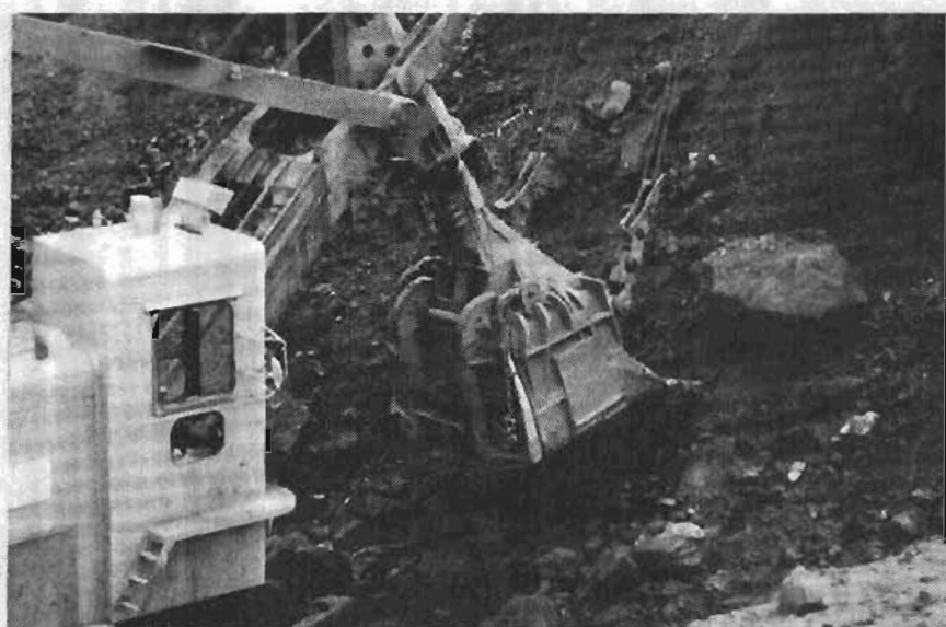
FIGURE F-4 HEATED SHOVEL BUCKET
