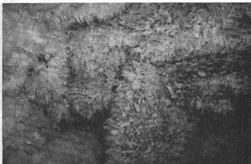
FIGURE H-2 ICE CRYSTAL BUILDUP ON MINE TIMBERS
