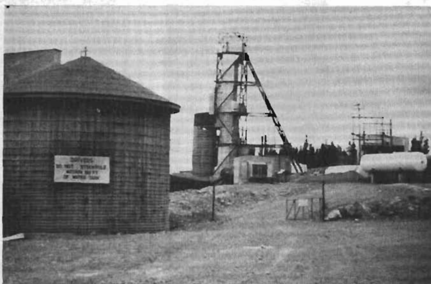
FIGURE J-1 MILL WATER STORAGE TANK (LEFT), HEADFRAME AND VENTILATION AIR HEATER (CENTER) AND PROPANE STORAGE TANK (RIGHT)
