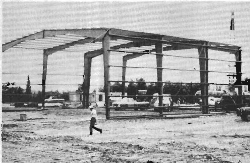
FIGURE I-2 ERECTION OF HEATED BUILDING FOR WINTER DRAGLINE CONSTRUCTION
