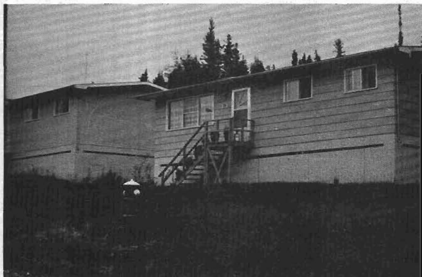
FIGURE E-3 HOMES ON PILE FOUNDATION, NOTE SKIRTING
