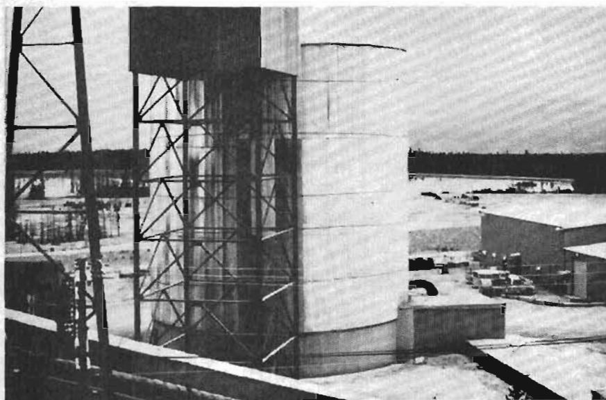
FIGURE J-3 HEATED AND INSULATED FINE ORE BIN
