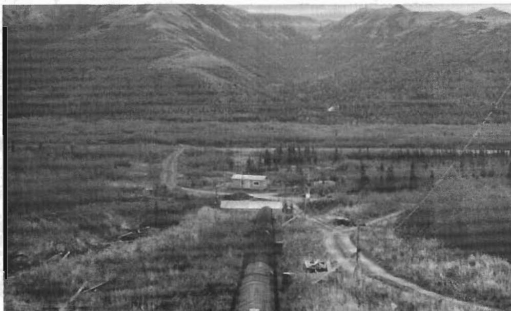
Figure 8. The 500 KW hydroelectric plant at Nyak has a penstock 5 feet in diameter, 550 feet long with a 70 foot head.
