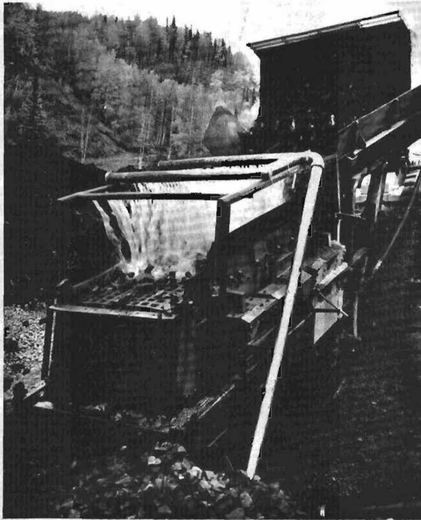
Figure 1. Shaking screen washing plant at Little Minook Creek, fed by a front end loader.
