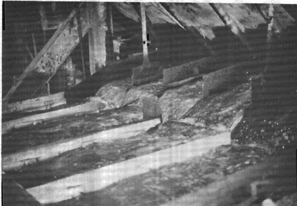
Figure 6. Tables receiving undersize material from trommel
