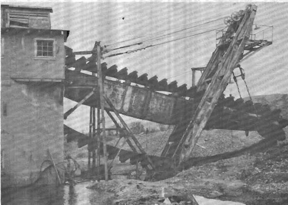
Figure 3. Bucket line on the dredge
