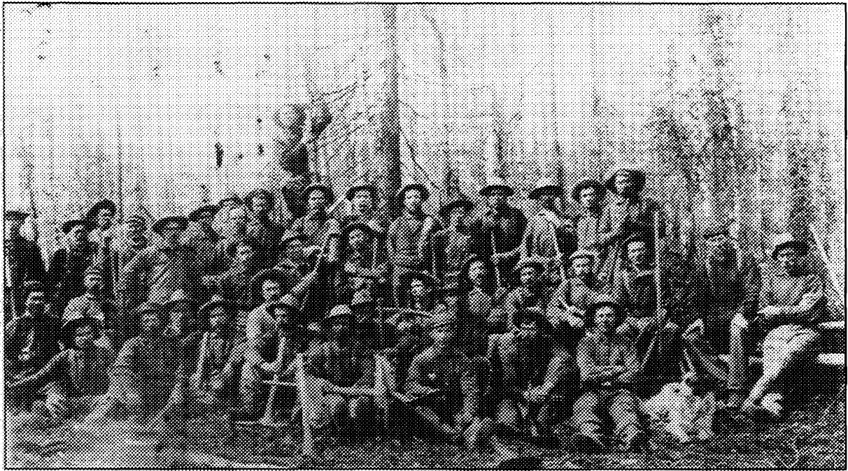
Figure 12. The so-called $3,000 ditching gang, Glen Gulch, 21 May 1902. Courtesy of the Herbert Heller Collection, University of Alaska Fairbanks. Accession Number 79-44-606N.
