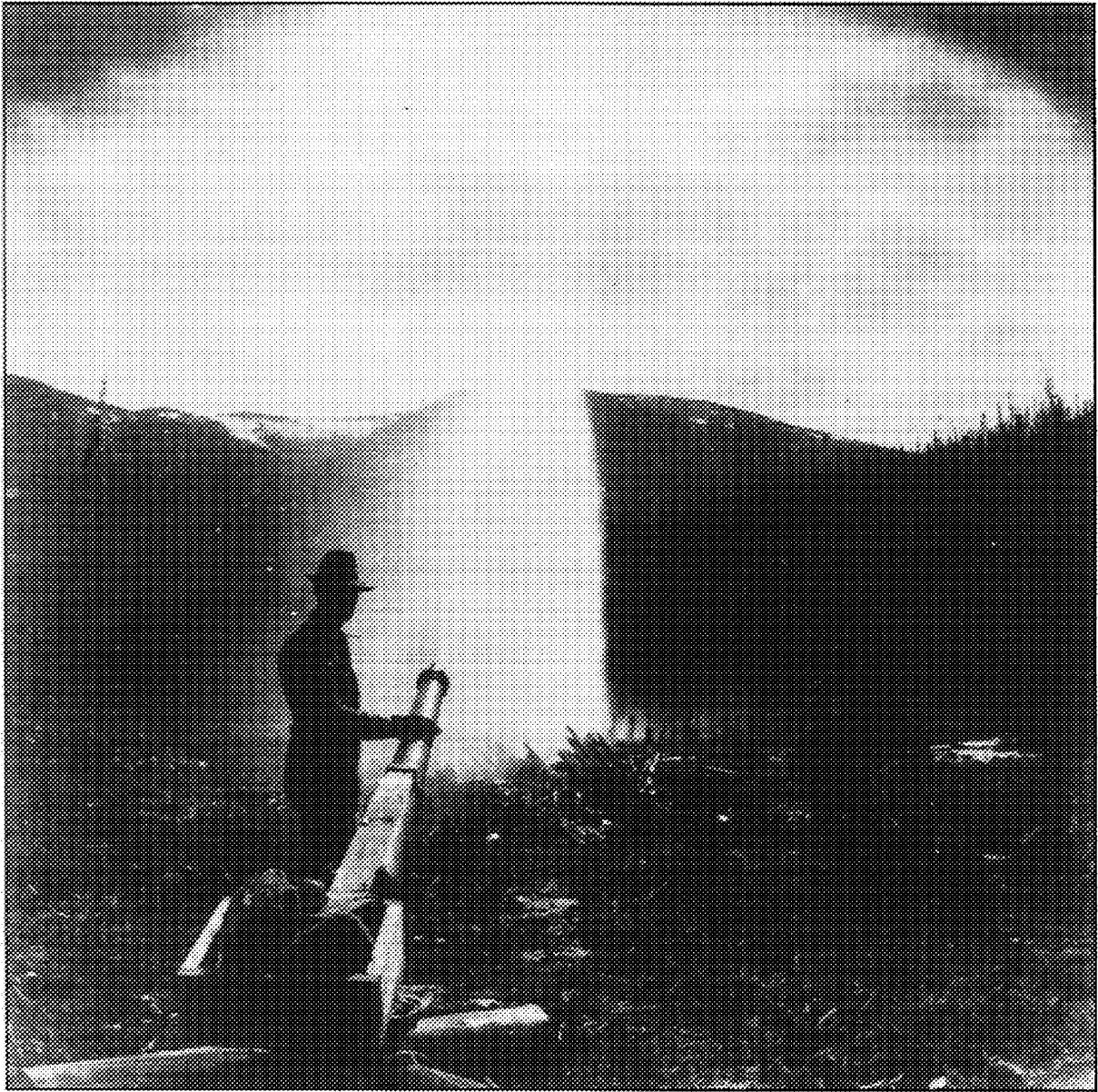
Figure 16. Hydraulicking on Hunter Creek, circa 1908. Courtesy of the William B. Ballou Collection, University of Alaska Fairbanks. Accession Number 72-47-5.
