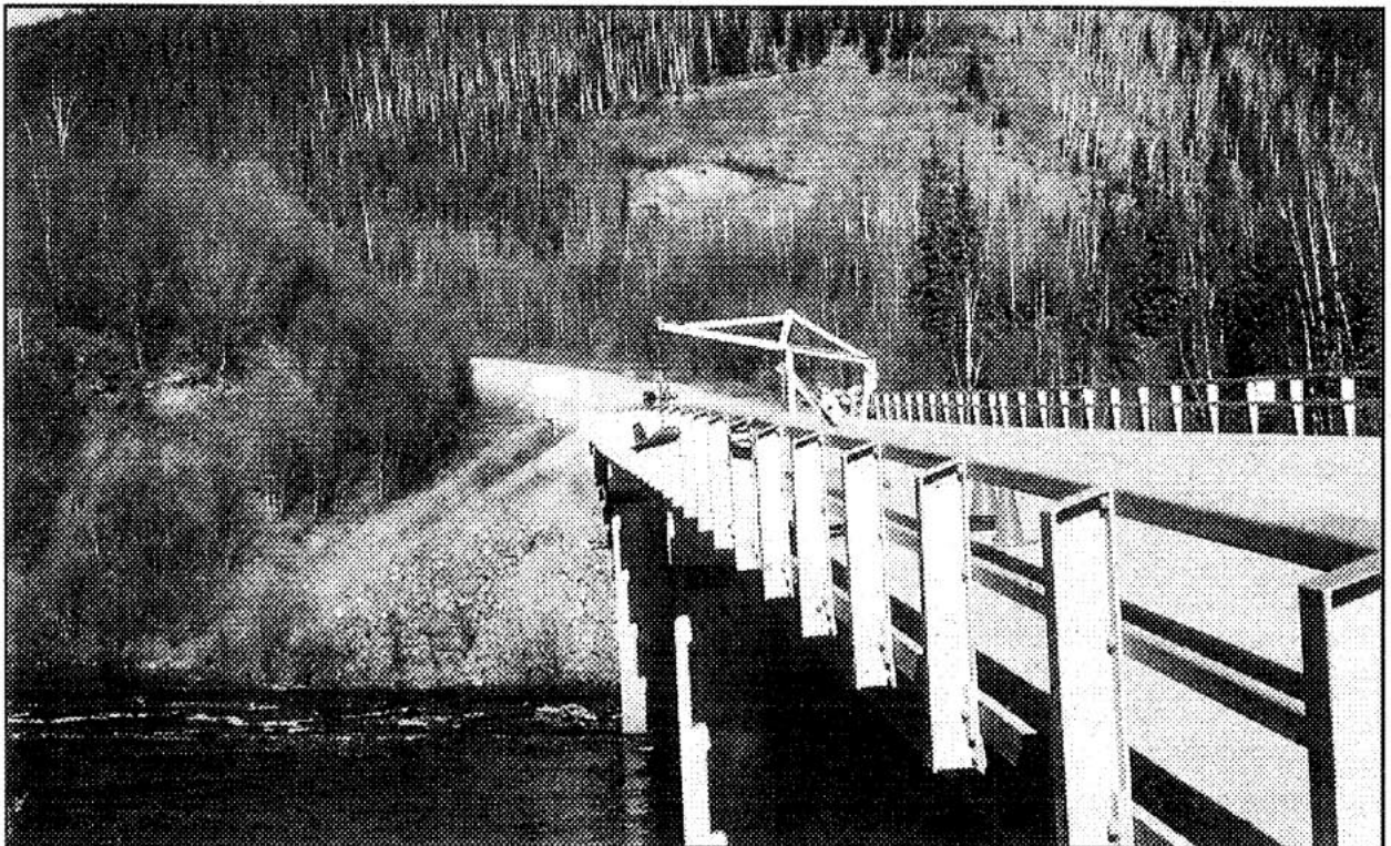
Figure 8. Measuring streamflow from the Taylor Highway bridge over South Fork.
