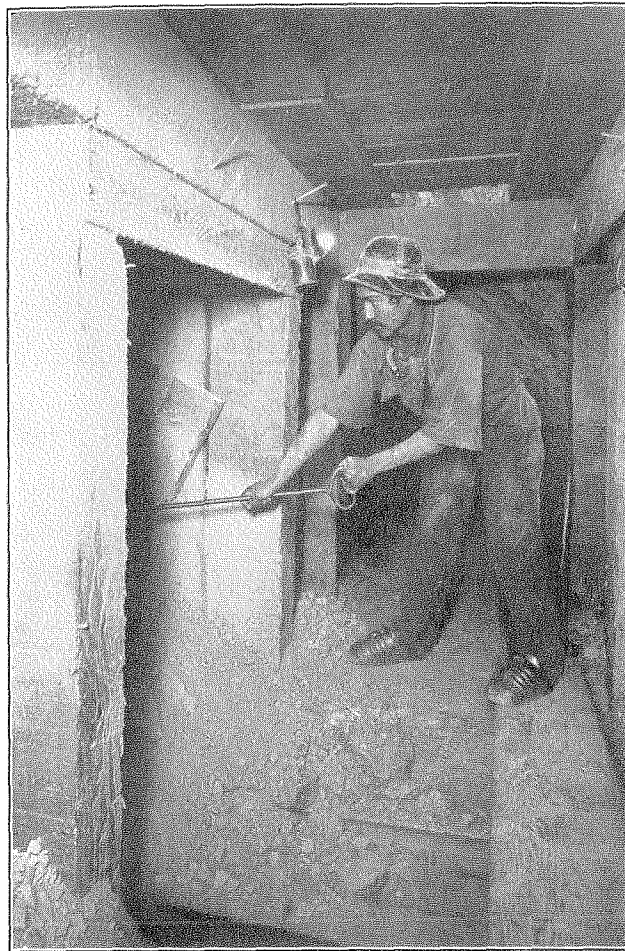
FIGURE 48.—Drawing ore from block-caving stope, Ray mine.
