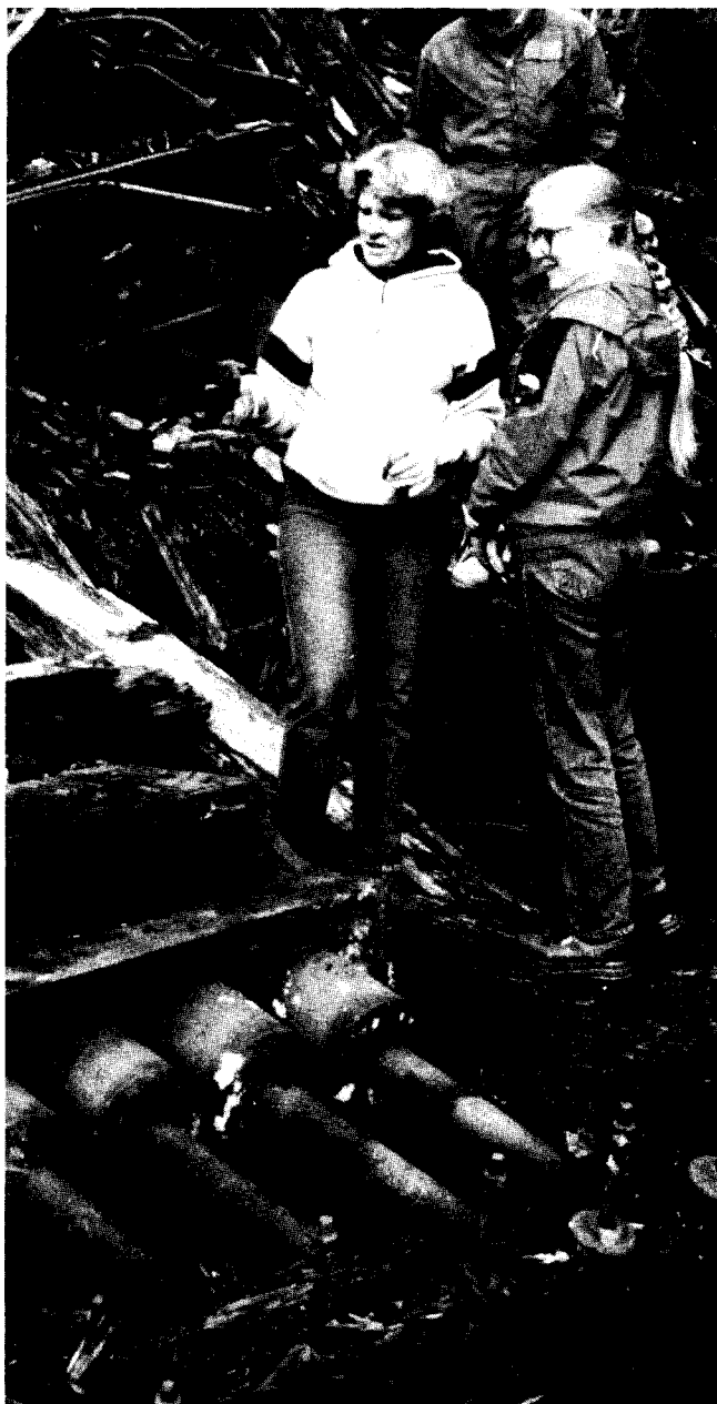
Figure D-201.—Remains of the Alaska Treasure 20-stamp mill which operated for only two weeks. Although extensively developed by 5,509 feet of workings, the Alaska Treasure prospect never produced more than a few hundred tons of ore because stamps were not able to recover the gold from the disseminated pyrite in the deposit.
