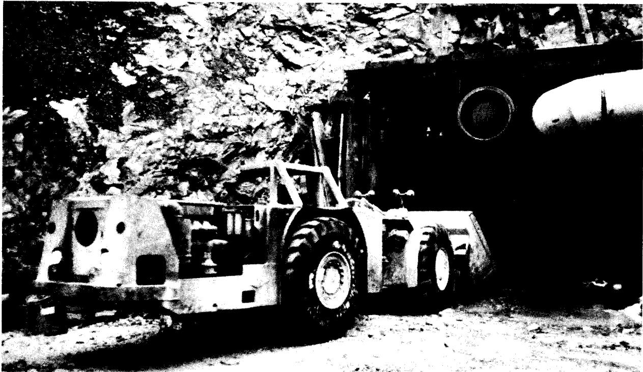
Figure D-23.—Portal of the new Kensington adit being driven by Echo Bay Mines and Coeur d'Alene Mines. This 5,300-ft adit undercut the Kensington deposit 1,200 feet below the old Kensington Tunnel.
