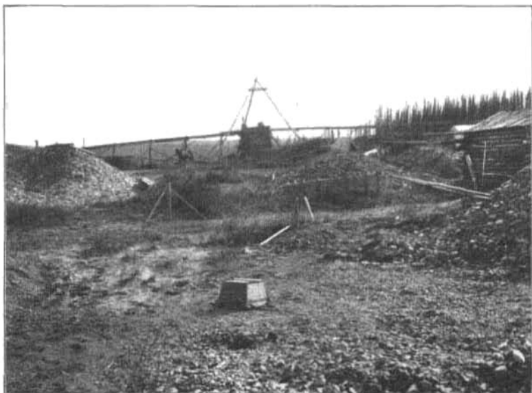
A. SHAFT AND HORSE HOIST ON CHICKEN CREEK.
