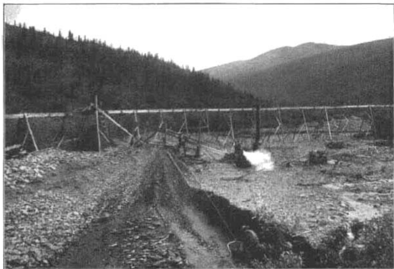
B. STEAM SCRAPER WITH BUCKET CONVEYOR AT MOUTH OF POKER CREEK.
