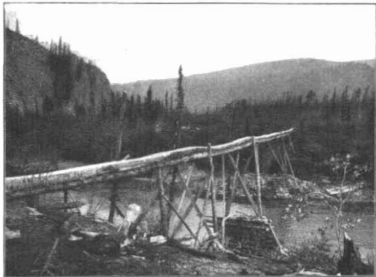
B. BRIDGE FOR CONVEYING WATER IN A CANVAS HOSE ACROSS SEVENTYMILE.
