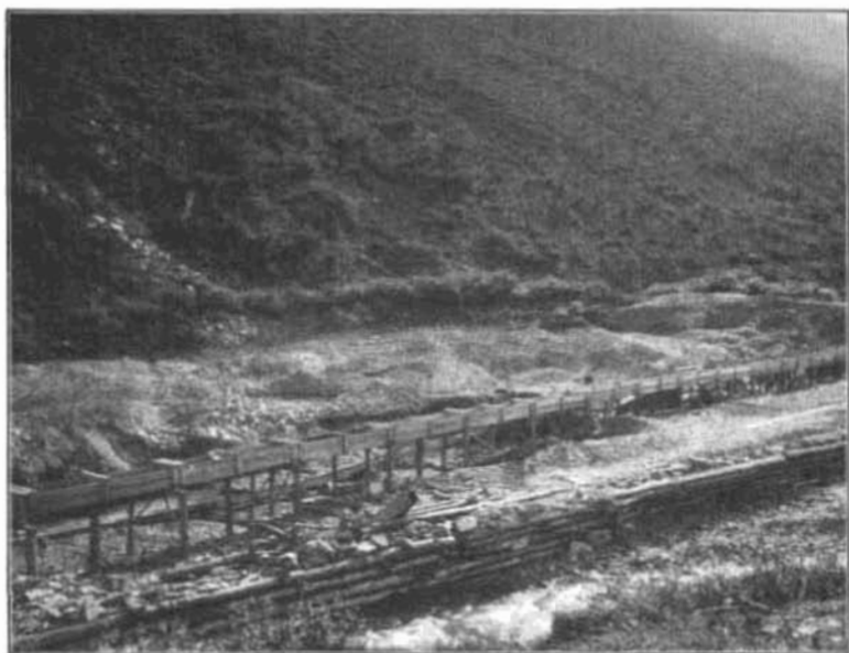
B. BED OF MASTODON CREEK WORKED BY OPEN CUTS.
