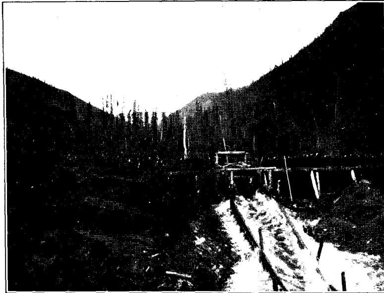
A. AUTOMATIC DUMP GATE DISCHARGING, CLAIM NO. 3 BELOW, LITTLE MINOOK CREEK.
