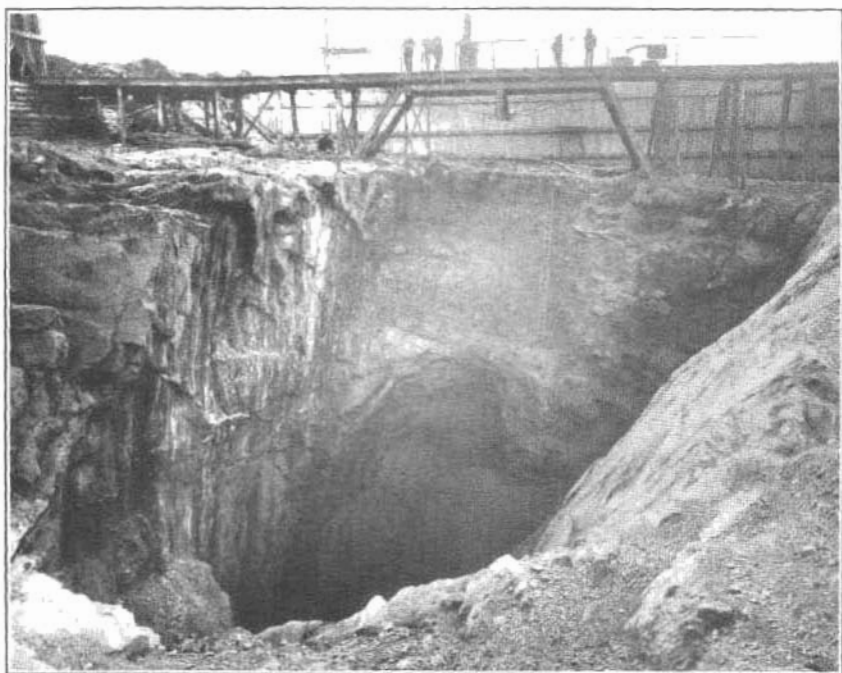
B. ORE BODY OF ELLAMAR MINE, EXPOSED IN GLORY HOLE WITHIN COFFERDAM.
