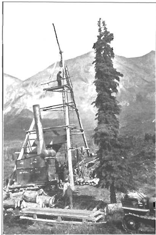
A. DIAMOND CORE DRILL AT NORTHWEST LOCATION ANTHRACITE RIDGE DISTRICT.
