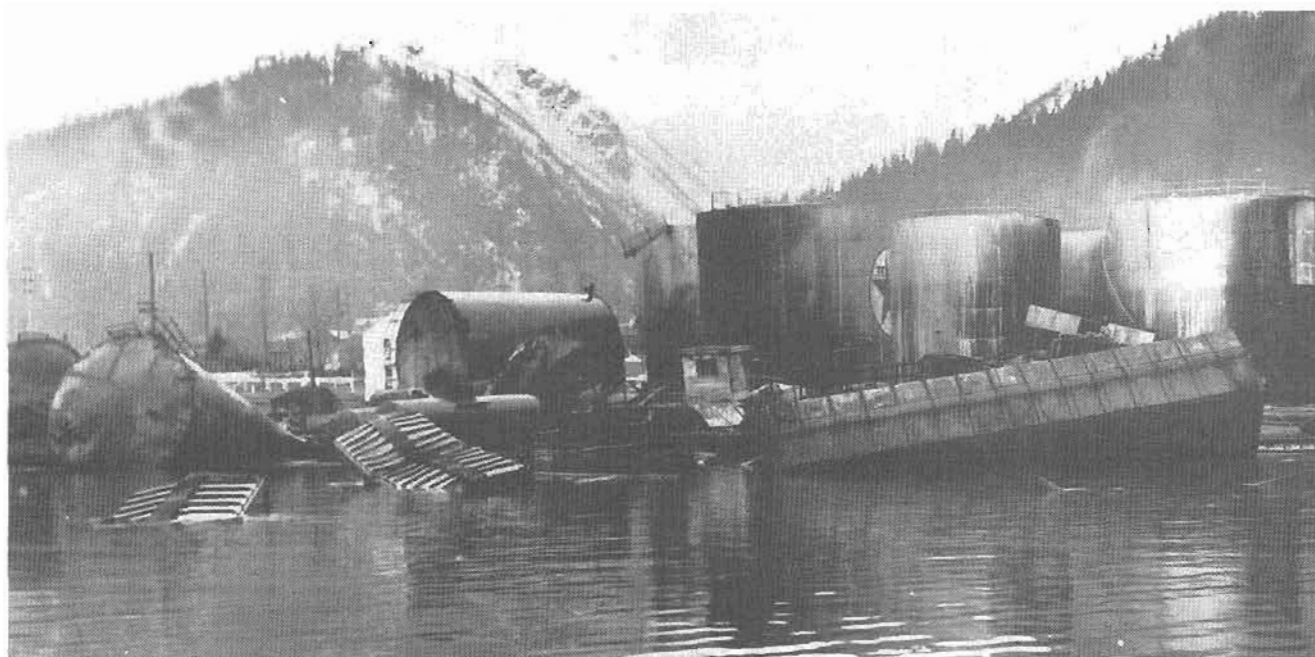
Figure 10. Landslide destruction of railroad and petroleum-storage facilities on the Seward waterfront (from Lemke, 1967).
