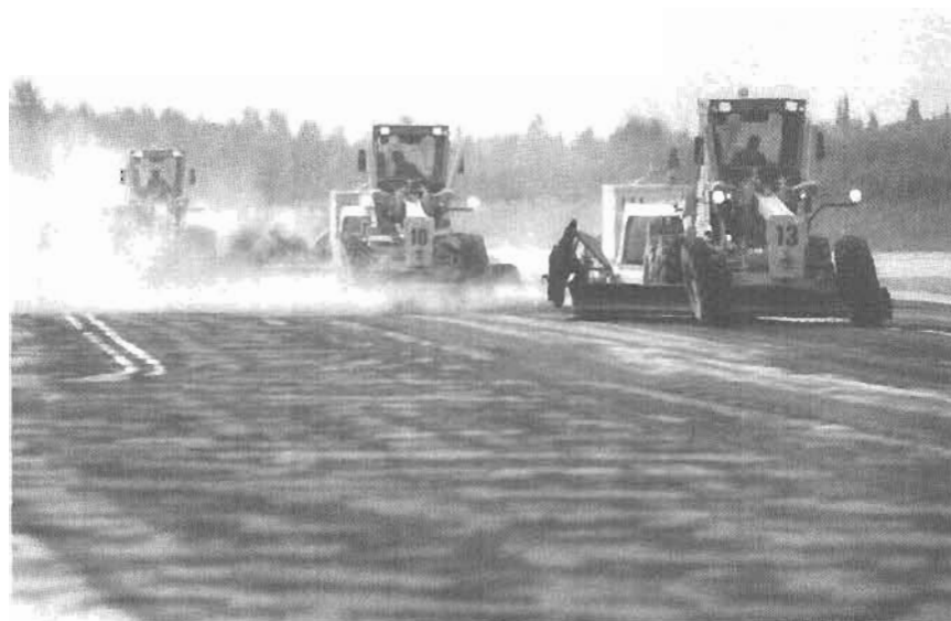
Figure 2. Road graders scrape ash from runways at Anchorage International Airport on August 19, 1992. Road scrapers could effectively move the ash only after it had been sprayed and dampened with water. However, too much water produced a slurry that could not be moved effectively. Dampened ash was scraped into furrows and then scooped up using front-end loaders. Some ash resuspended in the air would settle back onto runways and planes, and thus delayed aircraft cleanup. Photograph by Erik Hill courtesy of Anchorage Daily News.
