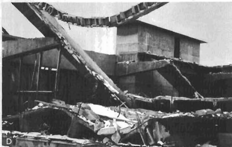
Figure 18. Photographs of destructive landslides and damage in ANCHORAGE. A , B , Graben at head of L Street landslide. C , Compressional ridge formed at toe of L Street landslide. D , Destruction by seismic shock of a partially complete concrete structure on unconsolidated deposits.
