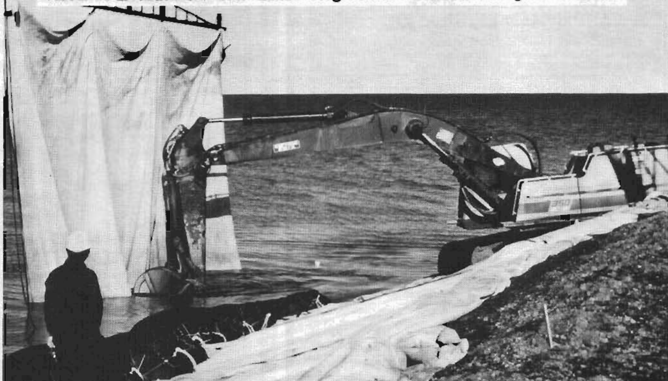
Construction of a gravel island for offshore drilling; the hanging cloth is a filter that protects the island's sediment base from erosion. The Minerals Management Service oversees this kind of activity.
