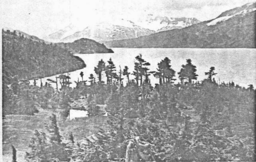
Figure 5. - View of Nellie Juan Lake from left abutment of damsite.
