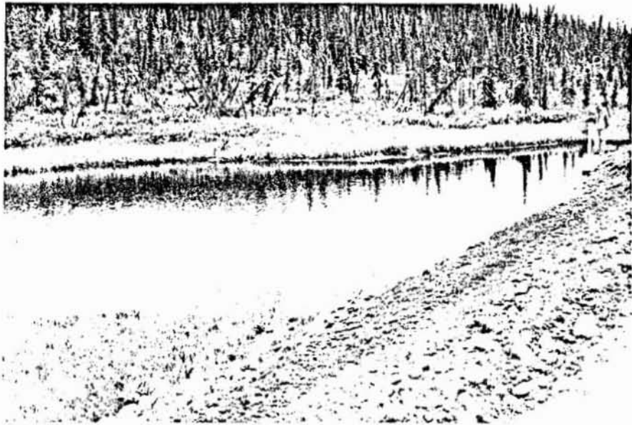
Figure 35. Pond formed since road construction (Site 100). June 25, 1975.
