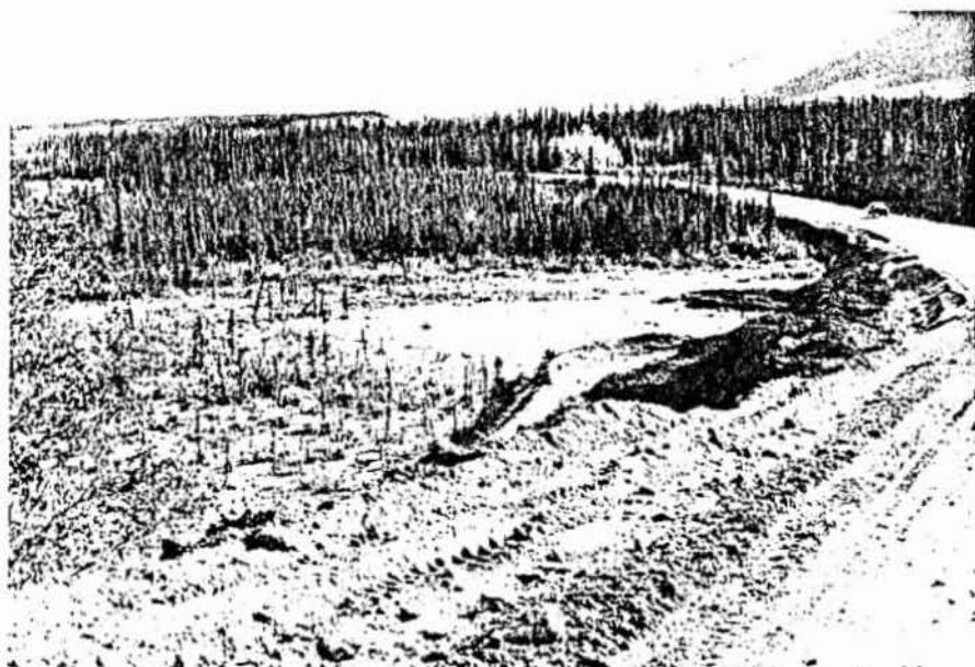
Figure 22. Siltation at base of road grade, Site 71. June 24, 1975.
