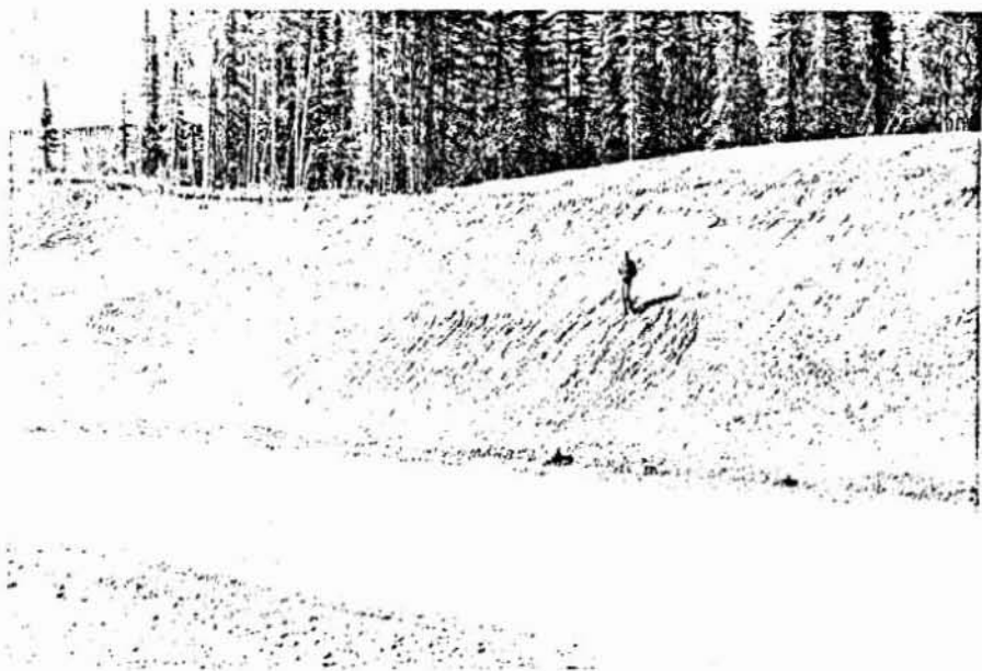
Figure 9. Road cut through ridge crest at Mile 11.3 (Site 27). Man is standing on contact between gravel and highly weathered bedrock. June 24, 1975.
