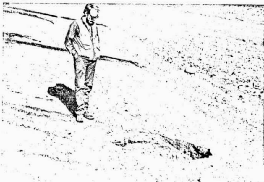
Figure 24. Piping in roadside ditch at Site 71. July 31, 1975.
