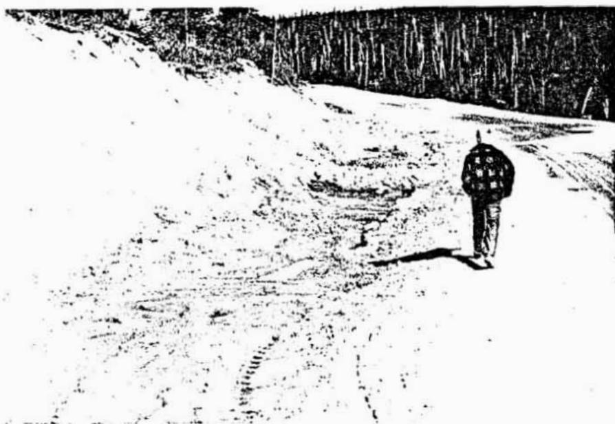
Figure 15. Wet, debris-filled ditch near Old Man Camp (Site 46). August 1, 1975.
