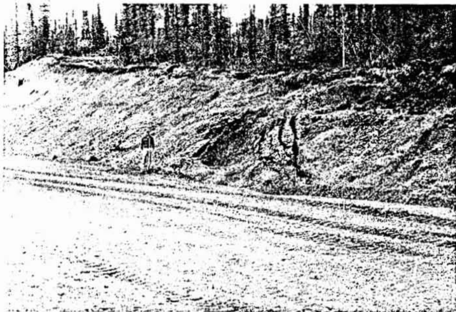
Figure 29. Thermokarst subsidence at Site 83. Subsidence is taking place beneath a berm of gravel which has been emplaced over face of road cut. June 25, 1975.
