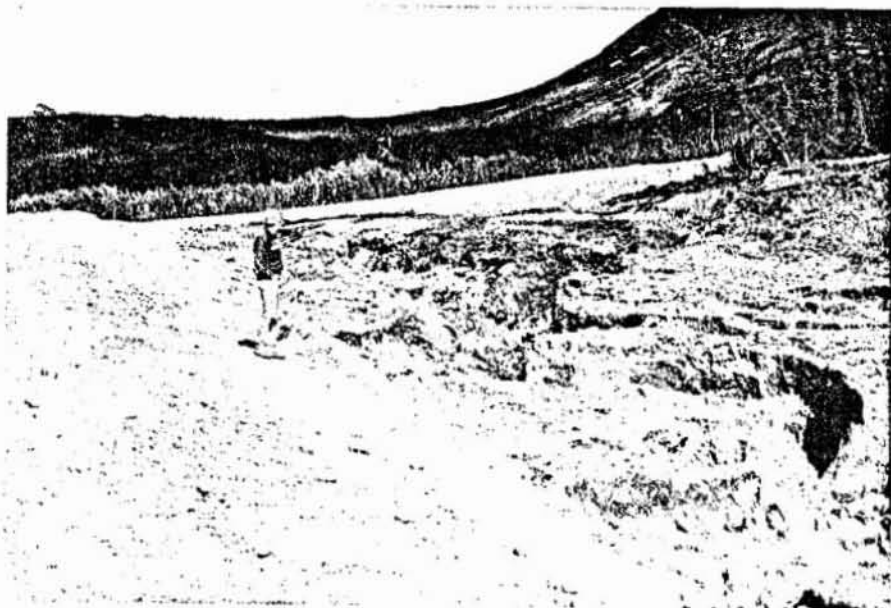
Figure 21. Gully erosion in roadside ditch at Site 71. June 24, 1975.
