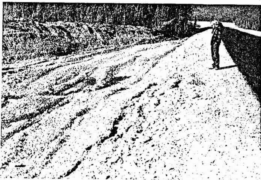
Figure 18. Sloughing of road edge into ditch at Site 58. August 1, 1975.
