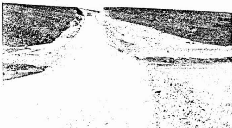
Figure 56. Road cuts into ice-rich muck above till and bedrock (Site 162). Disturbed areas on slope are mudflows and restraining structures. July 7, 1975.
