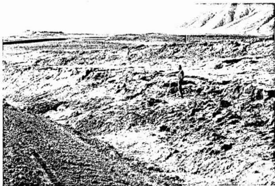
Figure 54. Slumping of eastern roadcut at north bank of Atigun River (Site 144). July 31, 1975.
