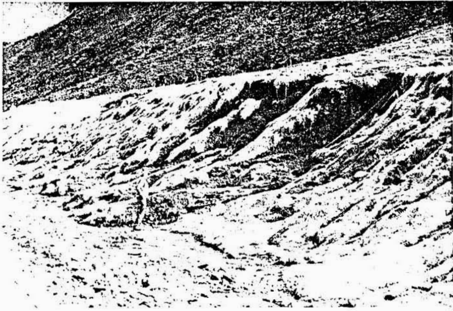
Figure 49. Active flows into eastern roadside ditch at Site 130. July 31, 1975.
