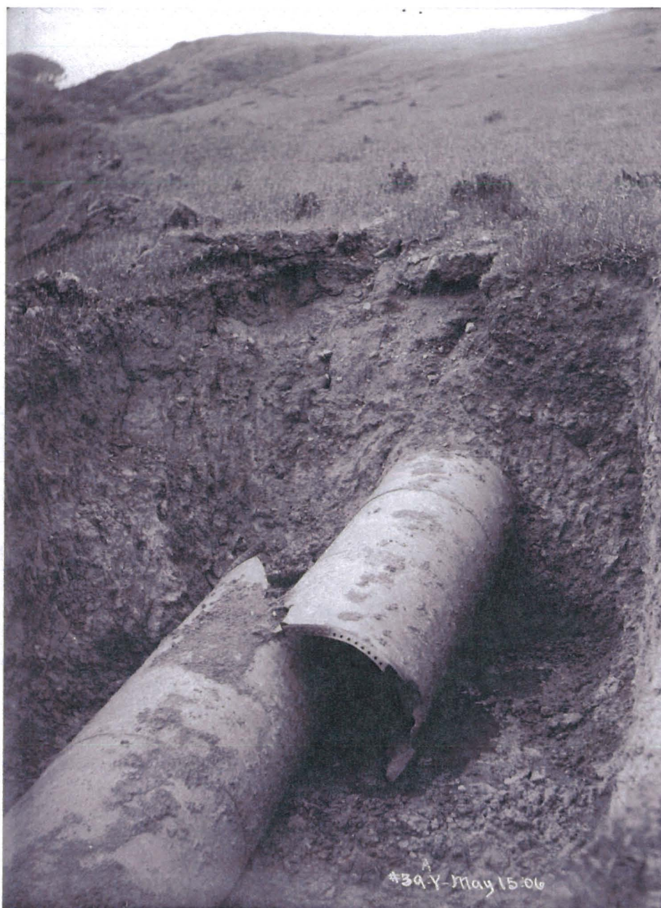
Figure 10. Damage to aqueduct by right-slip displacement on the San Andreas fault in 1906. The pipe, 76 cm in diameter, which crosses the fault from left to right, has been sheared and shortened. From Schussler (1906, photo 6), courtesy of San Francisco Water Department.
