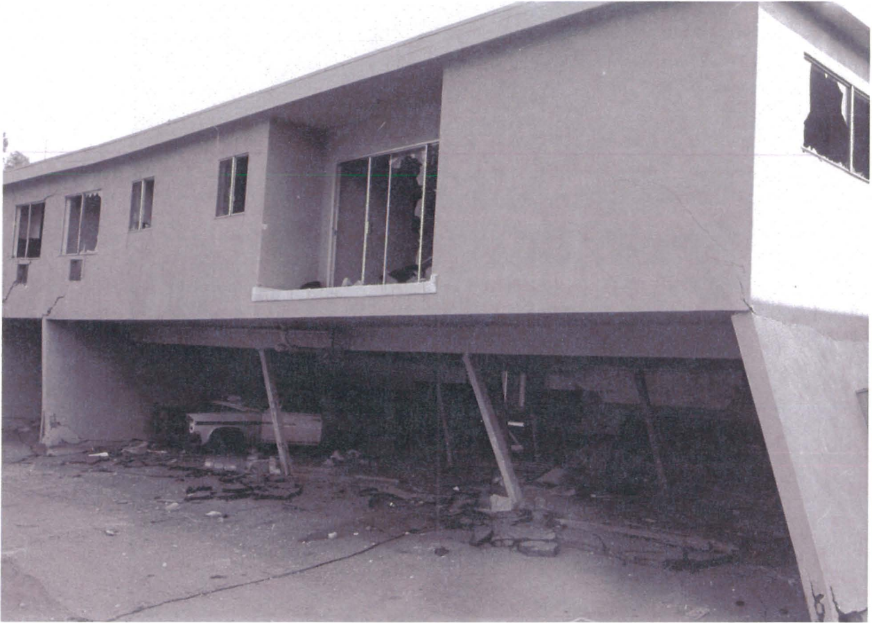
Figure 6. Damage to apartment house caused by about 2 m of reverse oblique-slip faulting during the Ms 6.6 1971 San Fernando, California, earthquake. The apartment had to be torn down. Photo by J. Schlocker.
