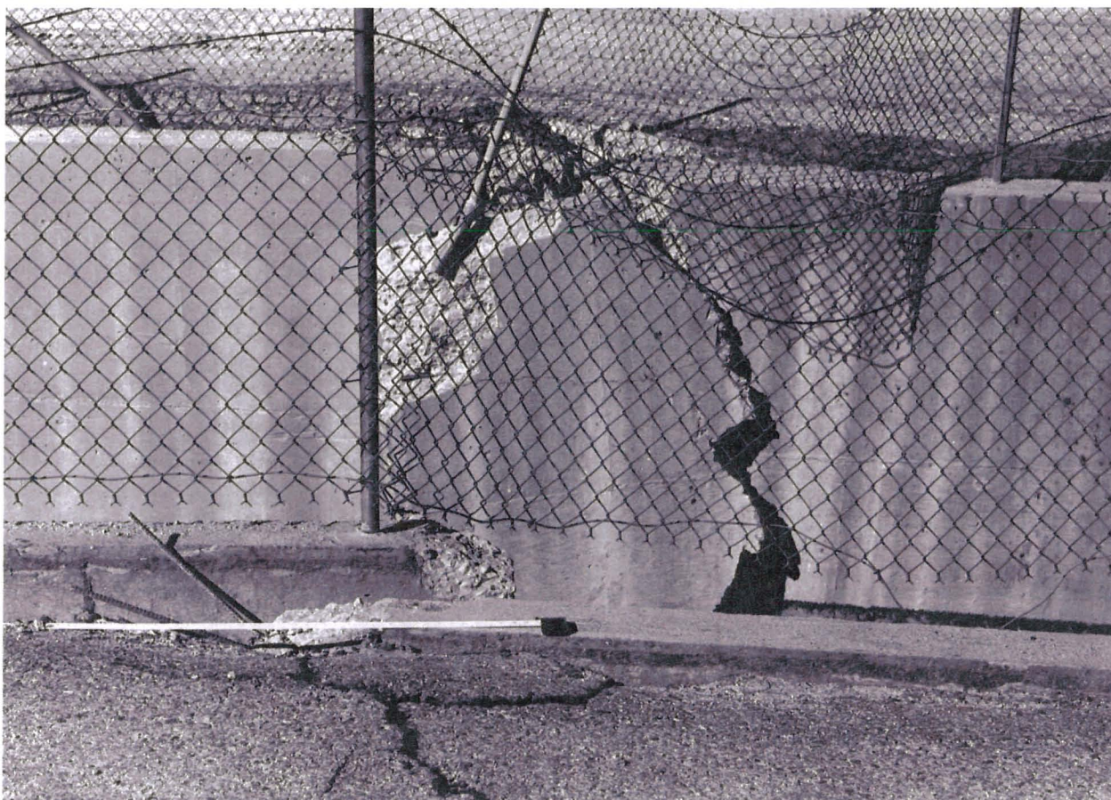
Figure 8. Compressional damage to reinforced concrete drainage channel caused by reverse-slip faulting in the 1971 San Fernando, California earthquake. East wall of channel (foreground) was broken and overlapped 0.9 m. Part of west wall (background) was broken and moved toward channel. This damage occurred about 75 m from the main fault trace. The channel and its damage are described by the Subcommittee on Water and Sewerage Systems (1973, p. 163-167). Photo by V.A. Frizzell.
