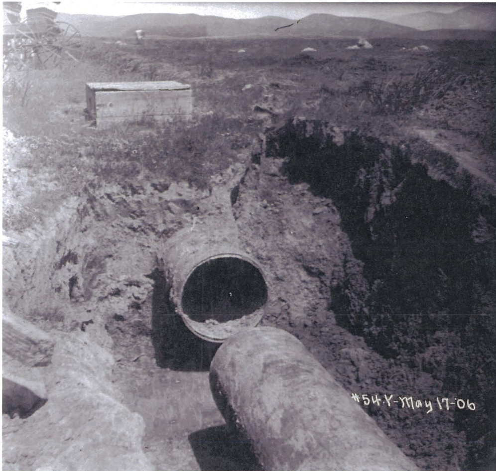
Figure 11. Aqueduct, which crosses the fault from right to left, was pulled apart about 1 m by right-slip displacement on the San Andreas fault, 1906. From Schussler (1906, fig. 7), courtesy of San Francisco Water Department.
