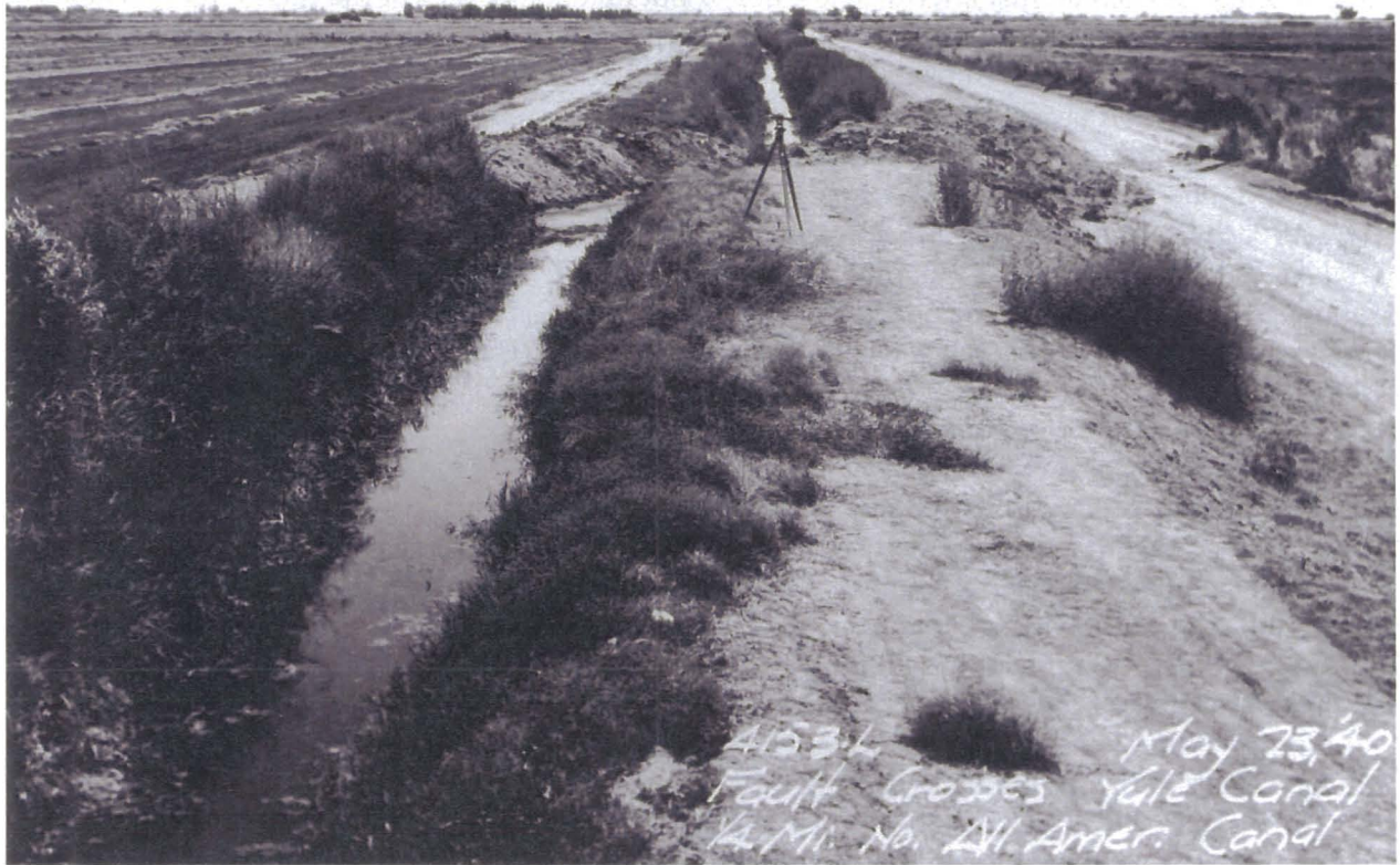
Figure 5. Canal displaced 4 m by strike-slip faulting in 1940, Imperial Valley, California. Photo courtesy of Imperial Irrigation District.
