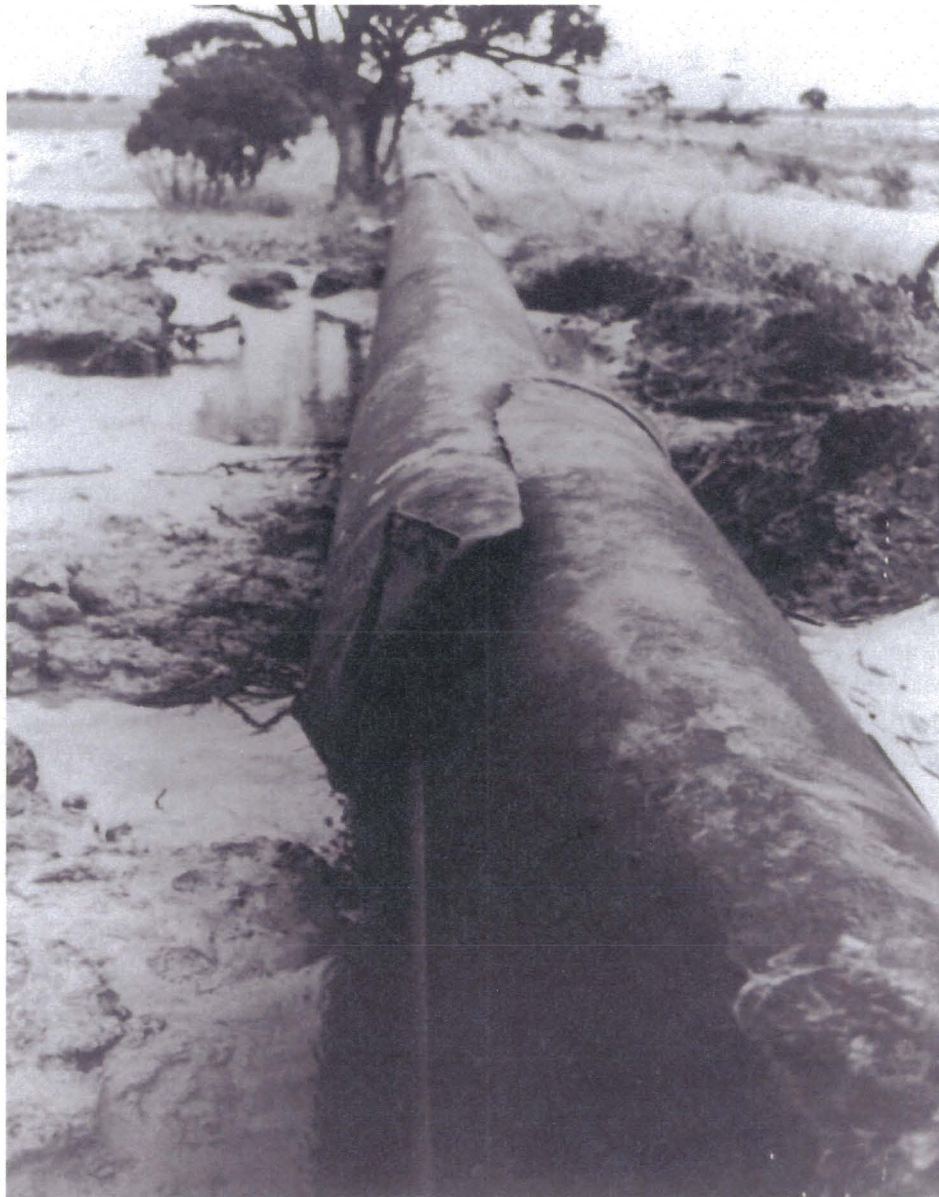
Figure 9. Compressional damage to one of a pair of water supply pipelines caused by reverse-slip faulting in Western Australia associated with an Ms 6.9 earthquake in 1968. Both pipes were telescoped 1.3 m, and reinforced concrete pipe supports were damaged on each side of the surface ruptures. For a distance of 400 m on one side of the fault and 1.2 km on the other side the pipe was shifted with respect to its supports. From Gordon and Lewis (1980, p. 22-23, fig. 9), courtesy of Geological Survey of Western Australia.
