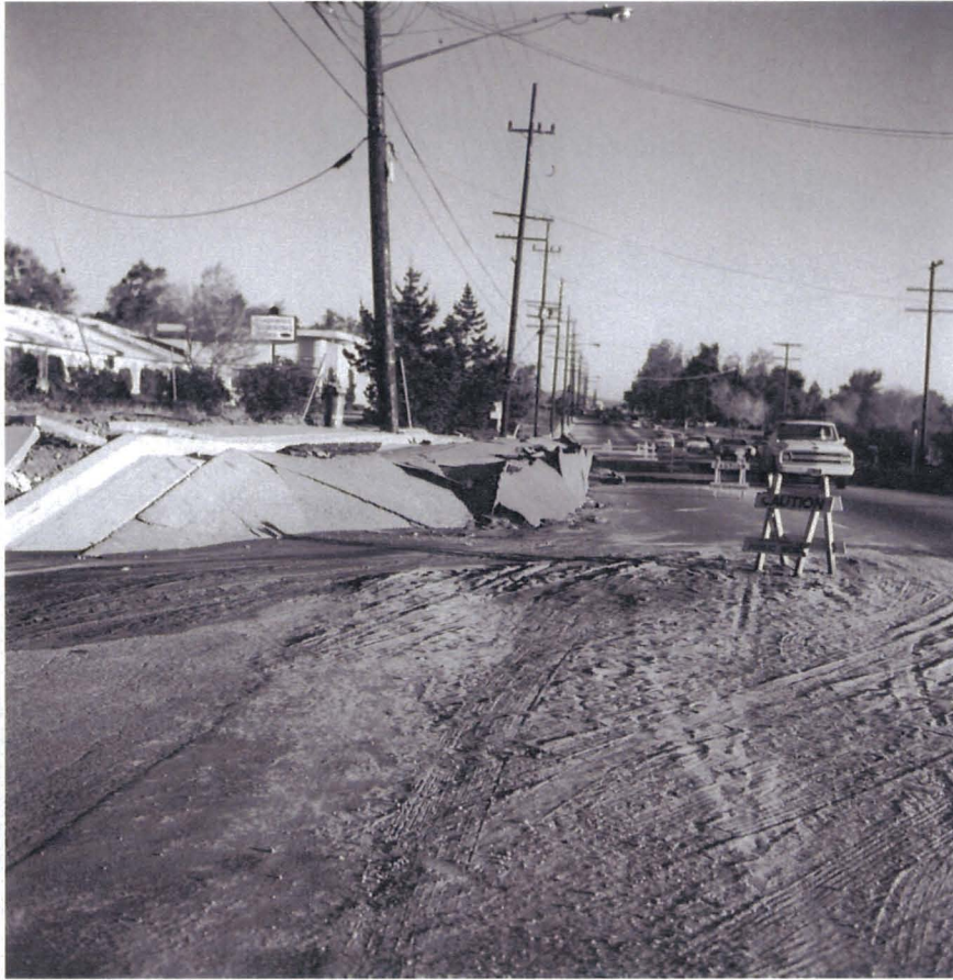
Figure 7. Damage to sidewalk, curb and pavement caused by 1.5 m of reverse-slip faulting, San Fernando, California, 1971. The nursing home on left was severely damaged by the faulting and had to be torn down. Photo by R. E. Wallace.
