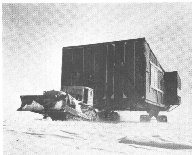
FIGURE 90.—Pump section of mobile rig on move from South Barrow test well 4 to Barrow camp, 19 April 1950. Photograph by U. S. Navy.
