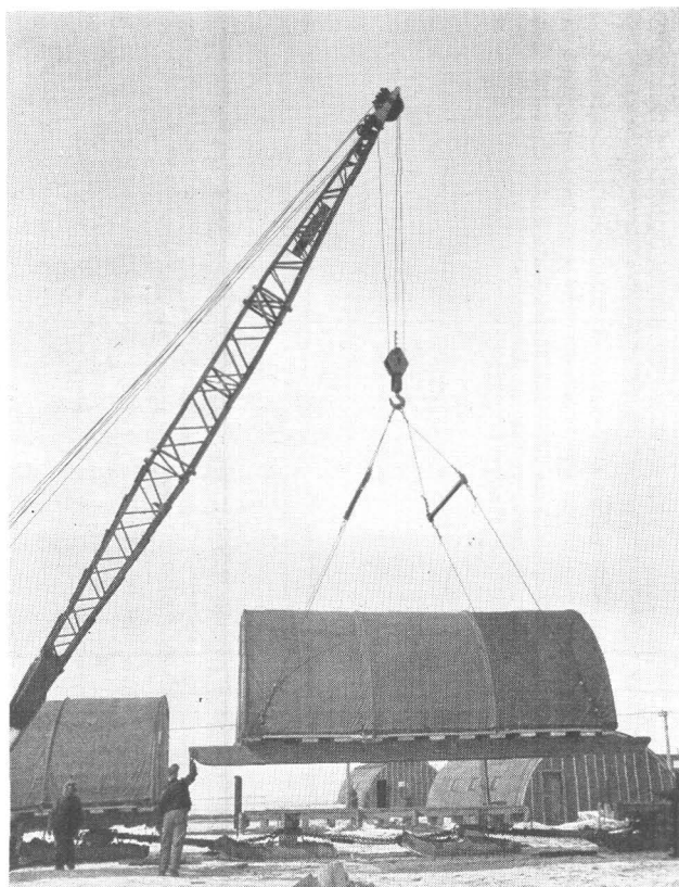
FIGURE 25.—Hoisting Jamesway huts onto Micheler sleds at Point Barrow for winter freighting, 7 May 1947. Photograph by U. S. Navy.
