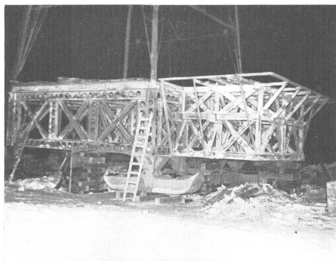
FIGURE 53.—Substructure for unitized Cardwell drilling rig with runners attached, 23 December 1949. Photograph by U. S. Navy.
