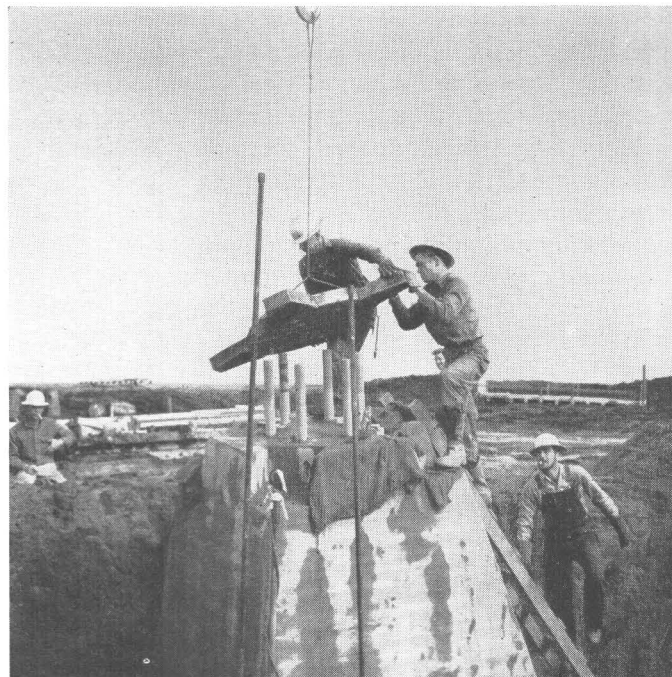
FIGURE 39.—Installing base plate for one of the legs of the Skull Cliff tower, 17 July 1947. Photograph by U. S. Navy.
