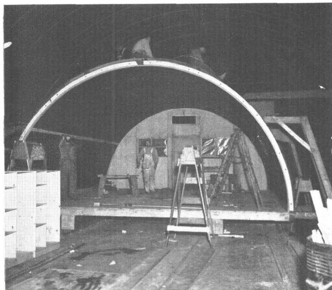
FIGURE 87.—Standard quonset hut under construction in carpenter shop at Barrow camp, April 1950. Photograph by U. S. Navy.
