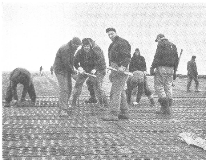
FIGURE 18.—Laying of marston mat on main runway of Barrow airfield, 8 June 1945. Photographs by U. S. Navy.
