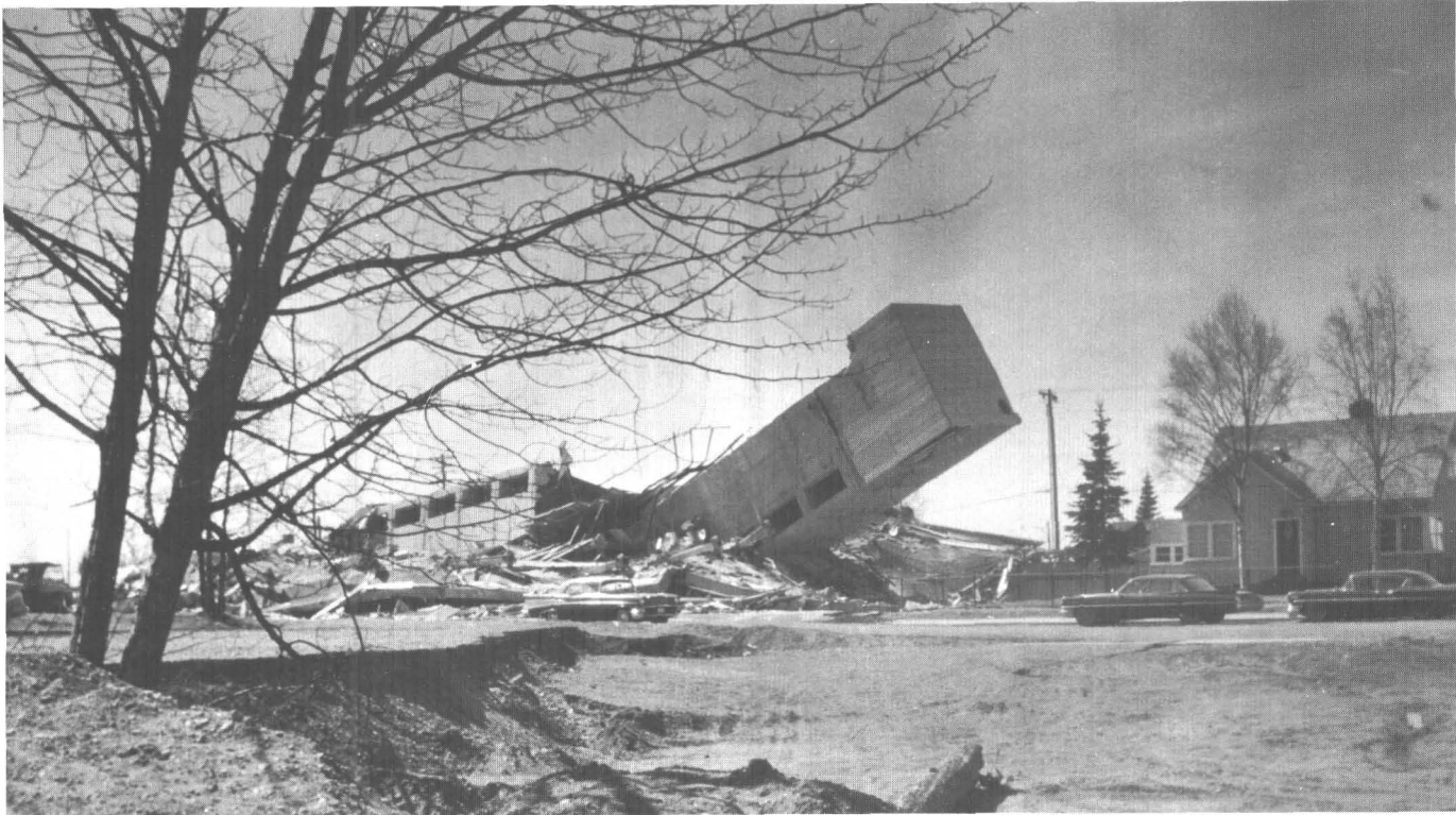
13.—Wreckage of six-story Four Seasons Apartment Building, Anchorage, Alaska. Canted elevator shaft at center. Large crack in foreground, filled in on M Street to restore traffic, passed beneath building.
