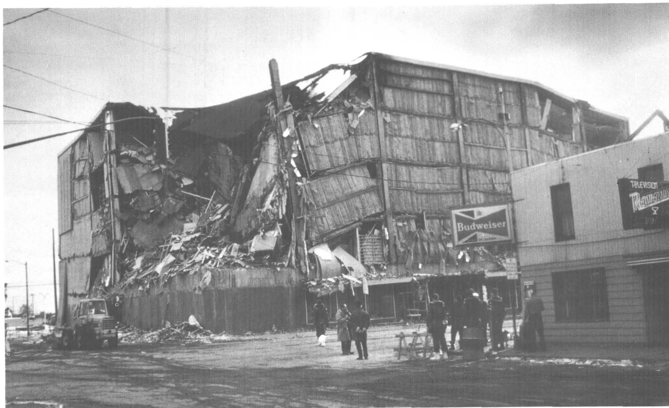
5.—Wreckage of Penney's department store, Fifth Avenue and D Street, Anchorage. Building failed after sustained seismic shaking. Most of rubble has been cleared from streets. Photograph by George Plafker.
