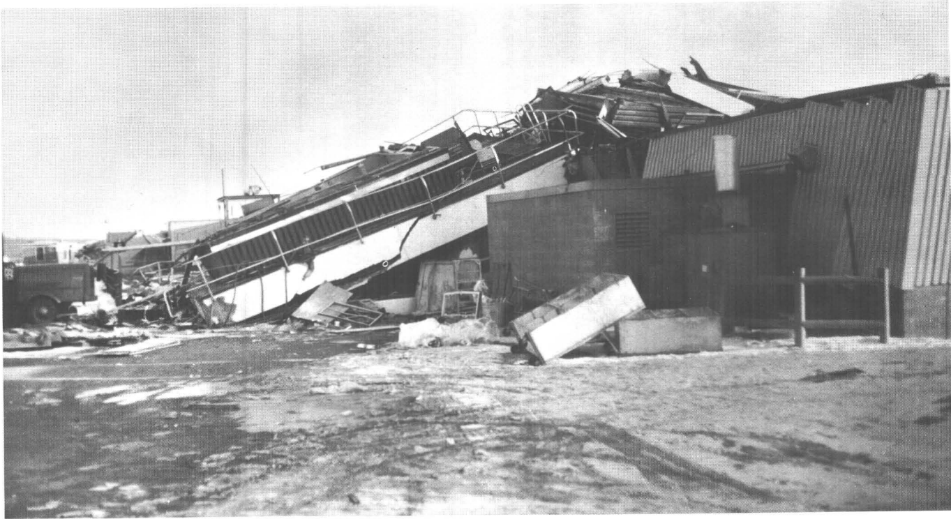
7.—Wreckage of control tower at Anchorage International Airport. Six-story tower failed under sustained seismic shaking. Photograph by George Plafker.
