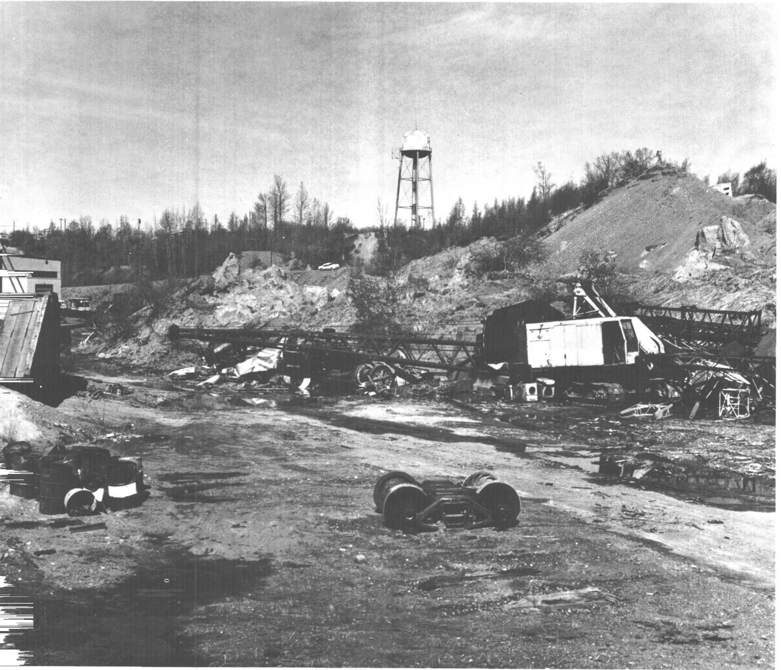
6.—Damage to yards of The Alaska Railroad, looking northwest, caused by earthflow at toe of Government Hill slide. Note undamaged water tank in background.
