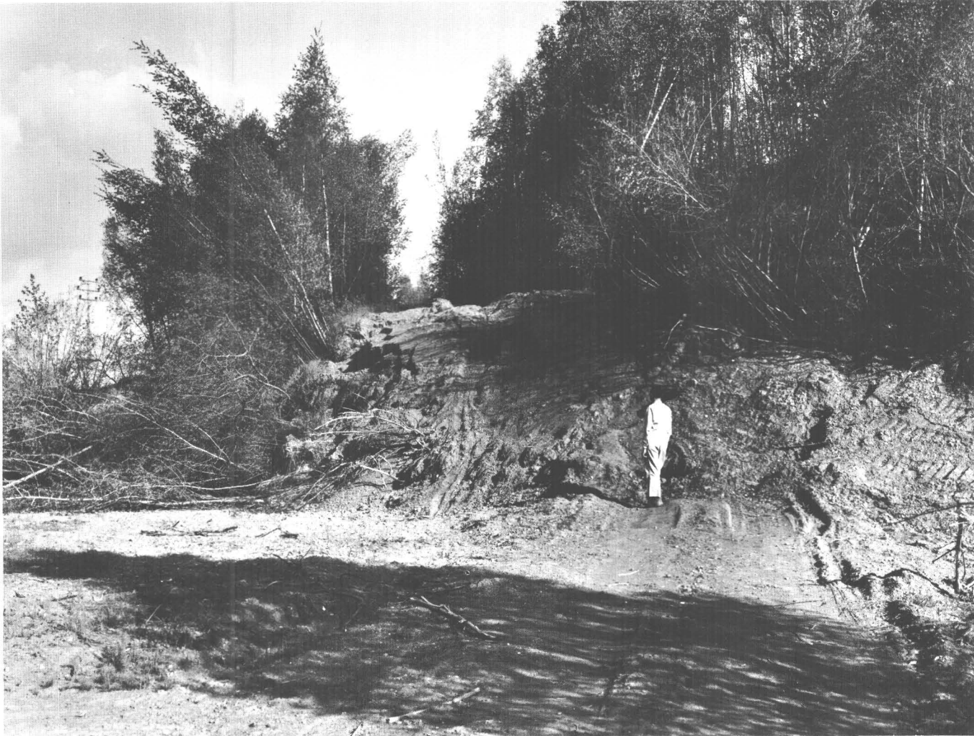
34.—Overthrust toe of Native Hospital slide. Road is bulged up and displaced about 12 feet laterally. Note overridden trees at left.
