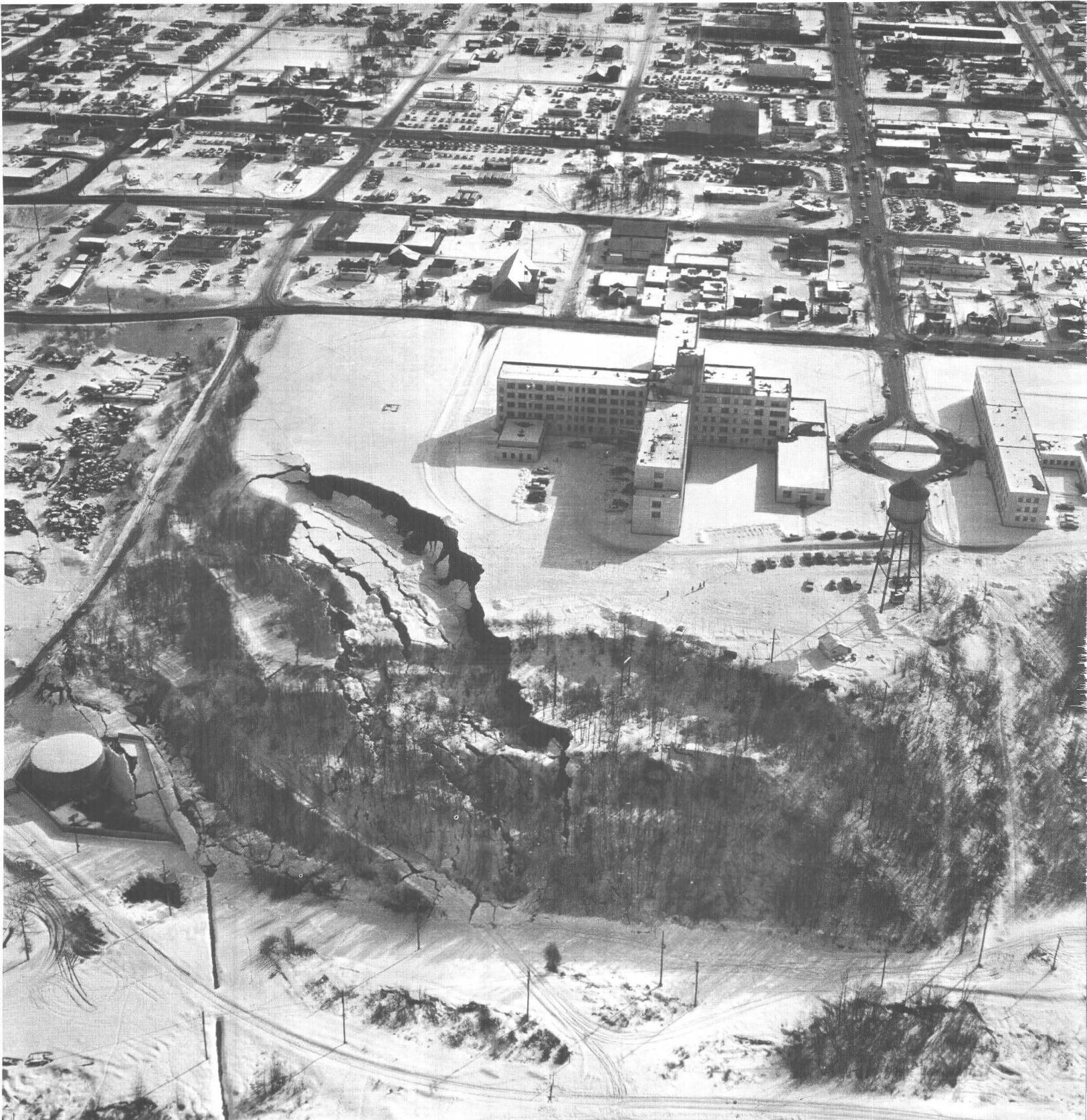
32.—Air view (looking south) of Native Hospital slide showing graben and pressure ridge. The scar of an older landslide is transected by the slide of March 27, 1964. Photograph by U.S. Army.
