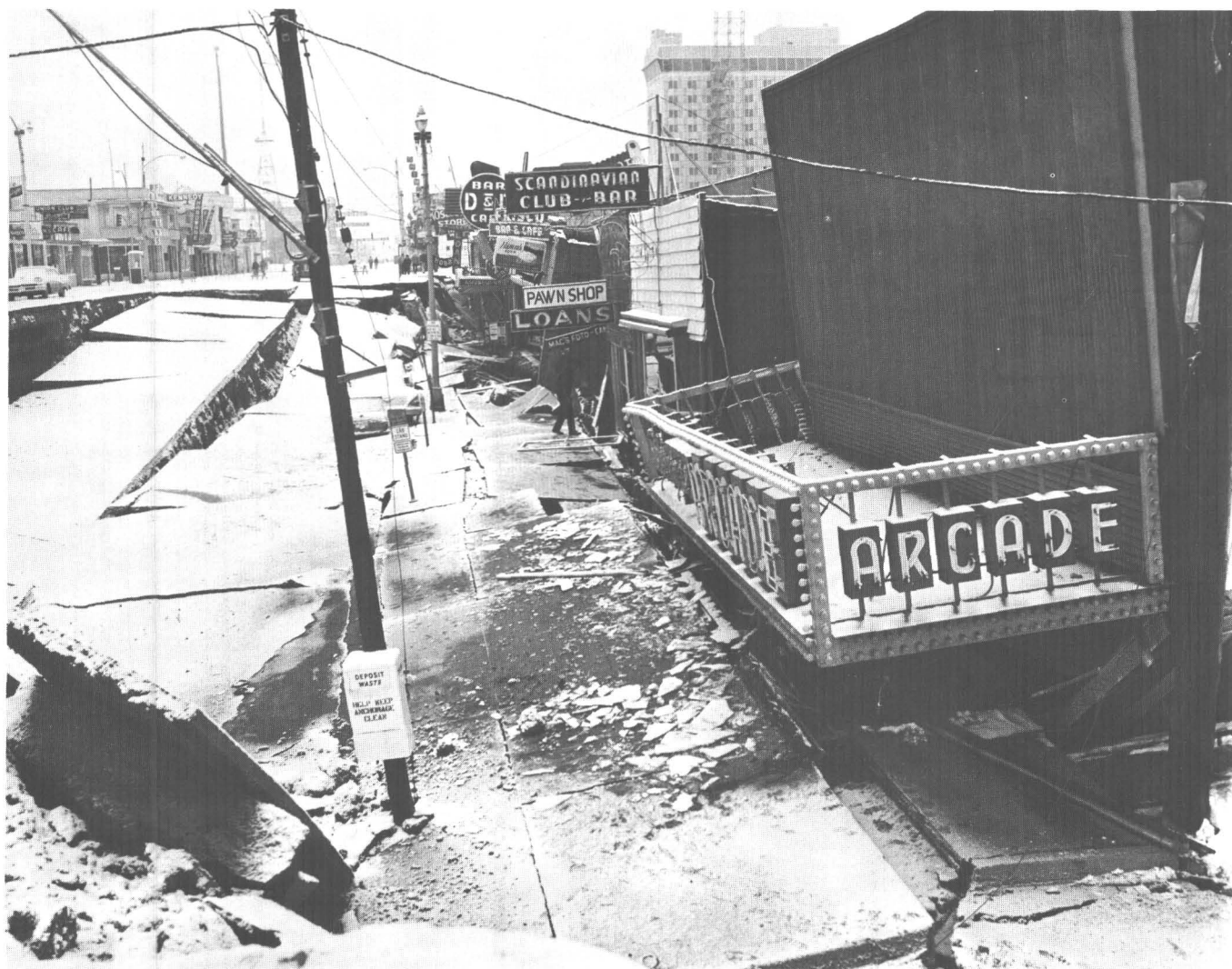
4.—View west along Fourth Avenue at head of landslide. North (right) side of street has collapsed into a graben. Vertical displacement is about 10 feet. Photograph by Mac's Foto, Anchorage, Alaska.
