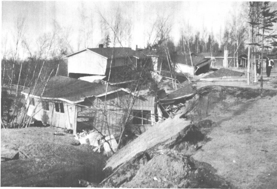
39.—Homes devastated by Turnagain Heights slide; deep within slide area, upper; at main scarp, lower. About 75 homes were destroyed.
