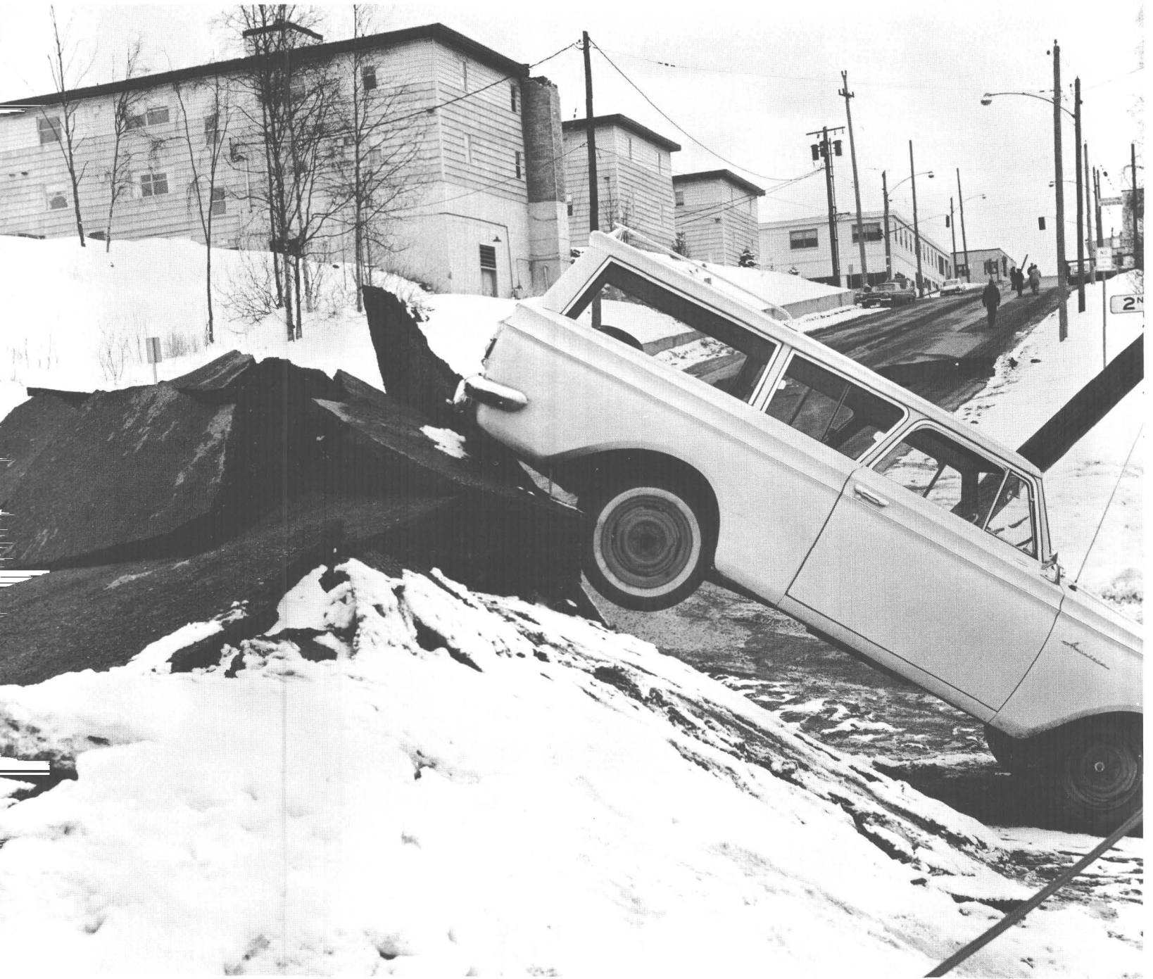
26.—Sharp-crested pressure ridge at Second Avenue and C Street, Anchorage. Probably caused by shallow translation of frozen surface layer. Note smaller pressure ridge in street part way up block and toppled chimney of building behind car. Photograph by Mac's Foto, Anchorage.
