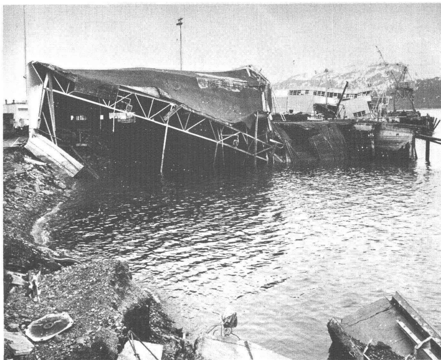
5.—Damage caused by water waves to old Alaska Railroad dock and facilities. Photograph by U.S. Army.
