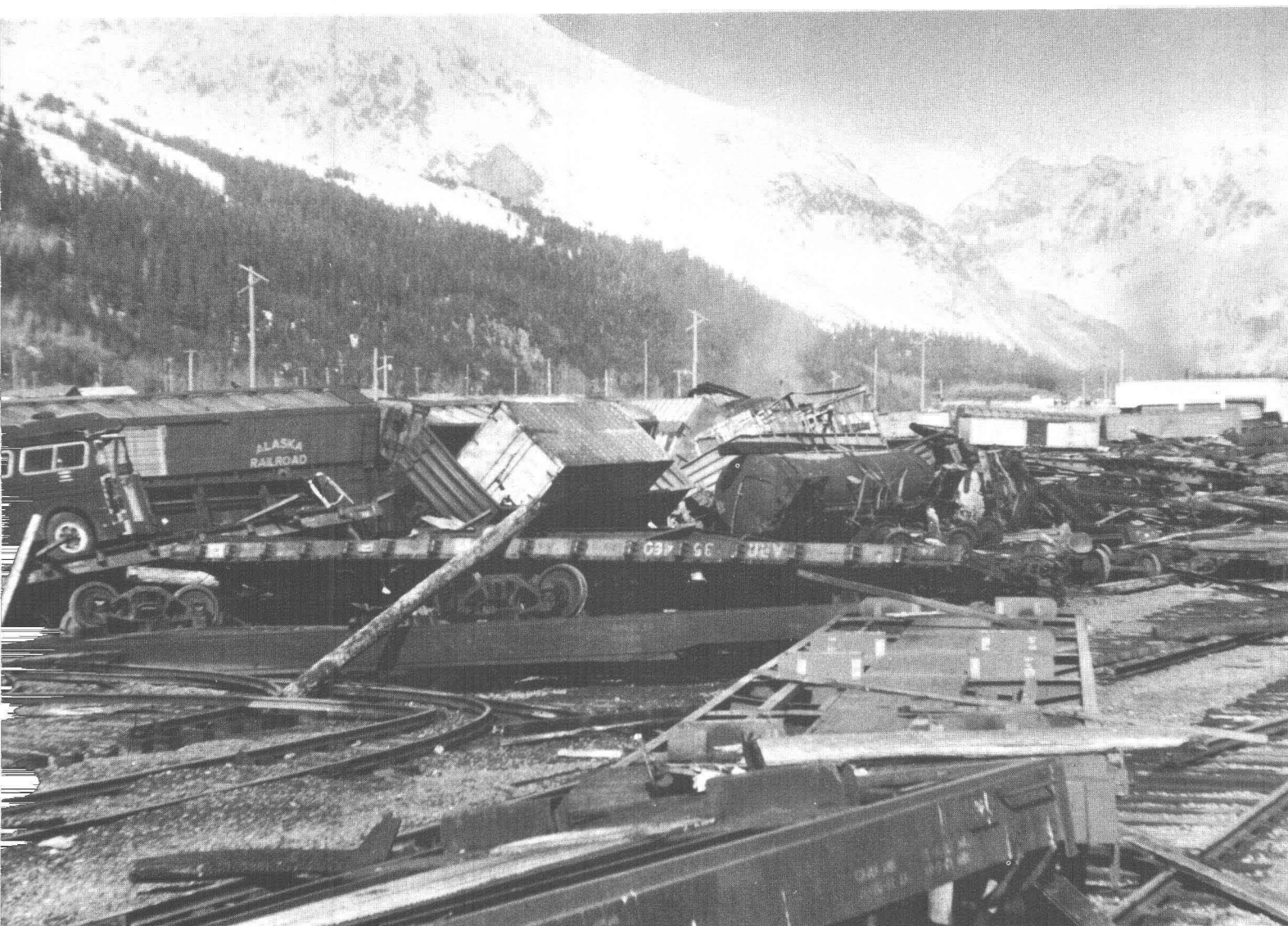
7.—Wave damage in the area of railroad marshalling yards.
