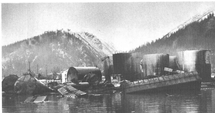
6.—Earthquake damage along Seward waterfront in area of Texaco, Inc., tanks. Photograph by U.S. Army.
