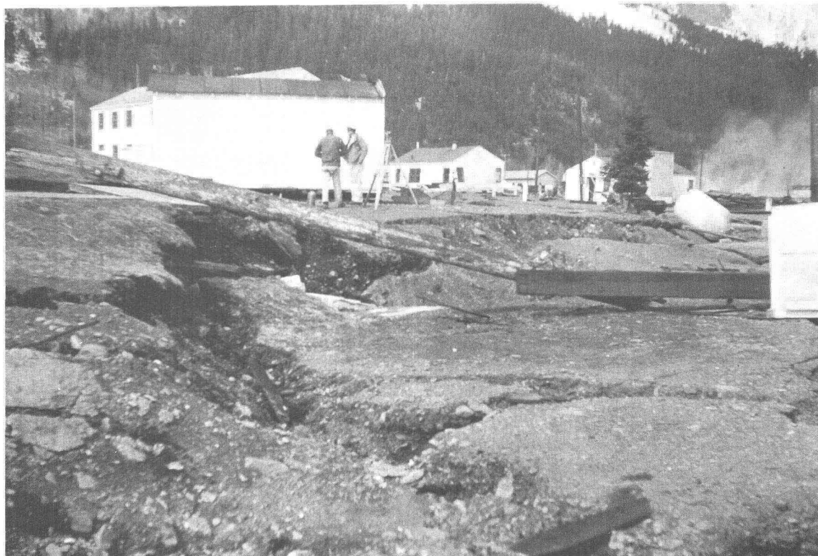
13.—Ground fracture near east end of A Street, about 100 feet from present shoreline, showing vertical displacement of about 4 feet. Downthrown side is toward Resurrection Bay.
