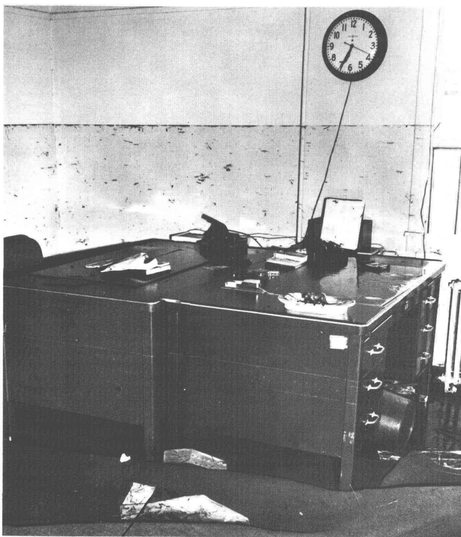
9.—Clock in the intelligence office, Kodiak Naval Station, showing time power failed at the station. Black watermark on the wall indicates maximum height of inundation. Photograph by U.S. Navy, March 29, 1964.
