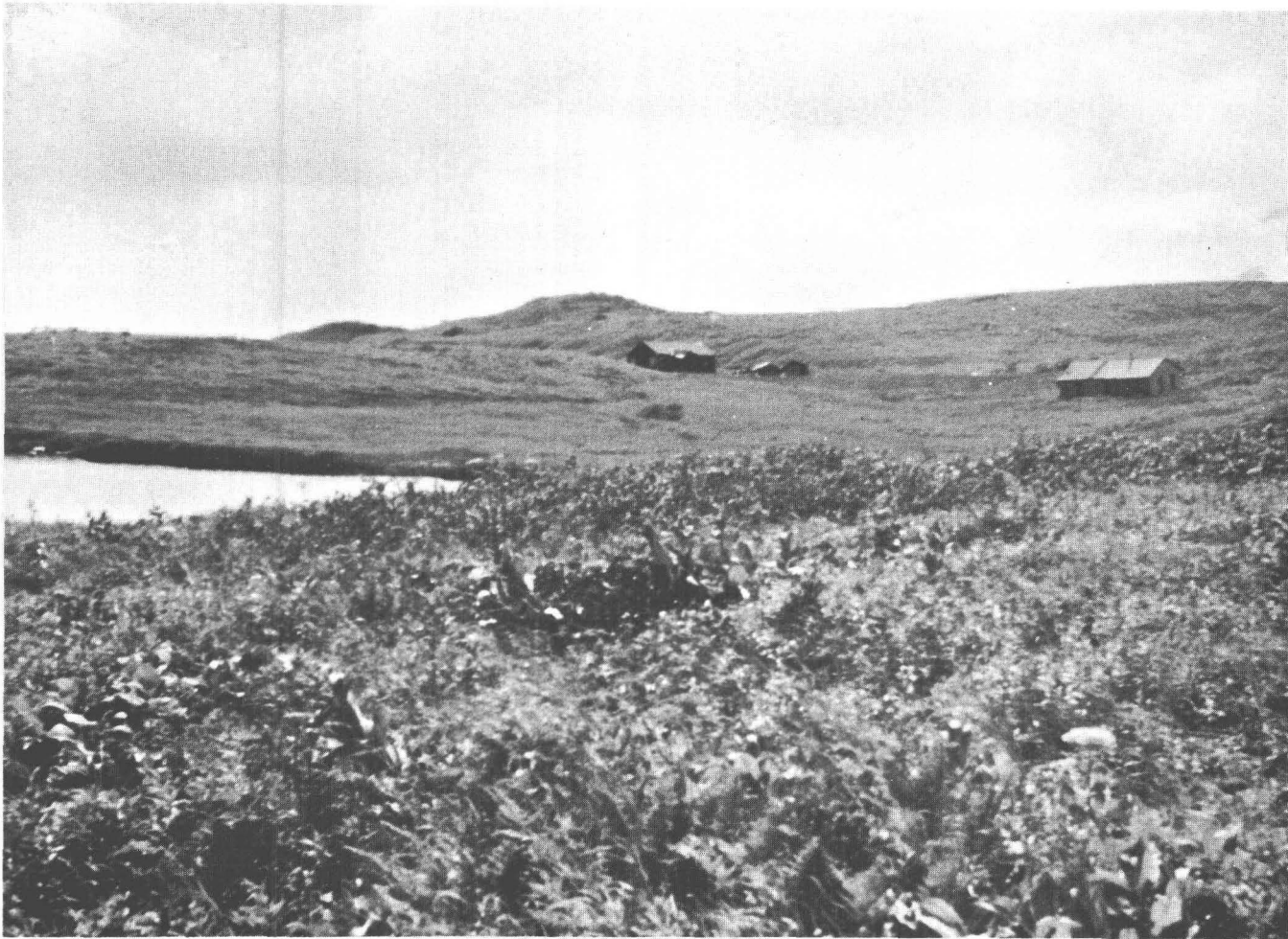
30.—Wood-frame houses that were floated inland from Kaguyak by seismic sea waves and deposited almost undamaged.
