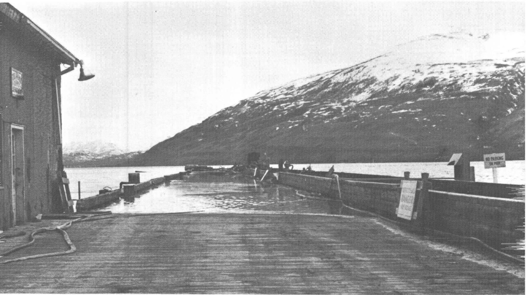
7.—Inundation of fuel pier during high tide at Kodiak Naval Station. Photograph by U.S. Navy, 12:59 p.m., April 12, 1964.
