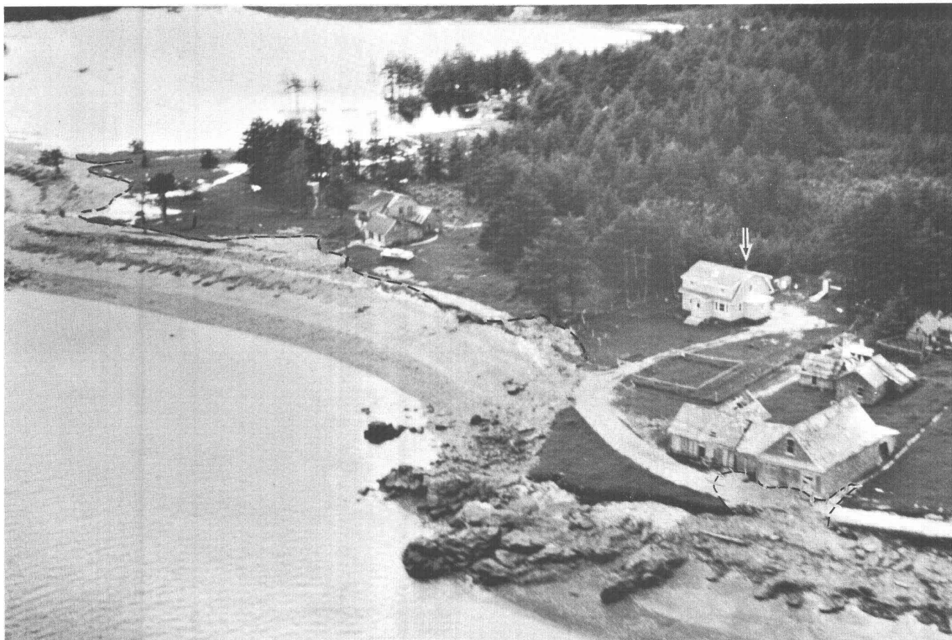
22.—Part of Afognak; note eroded road along coast, new beach berms (outlined by dashed line), and part of large lagoon ponded behind beach berm. The arrow points to undamaged brick chimney. Location of this view is shown on figure 21.
