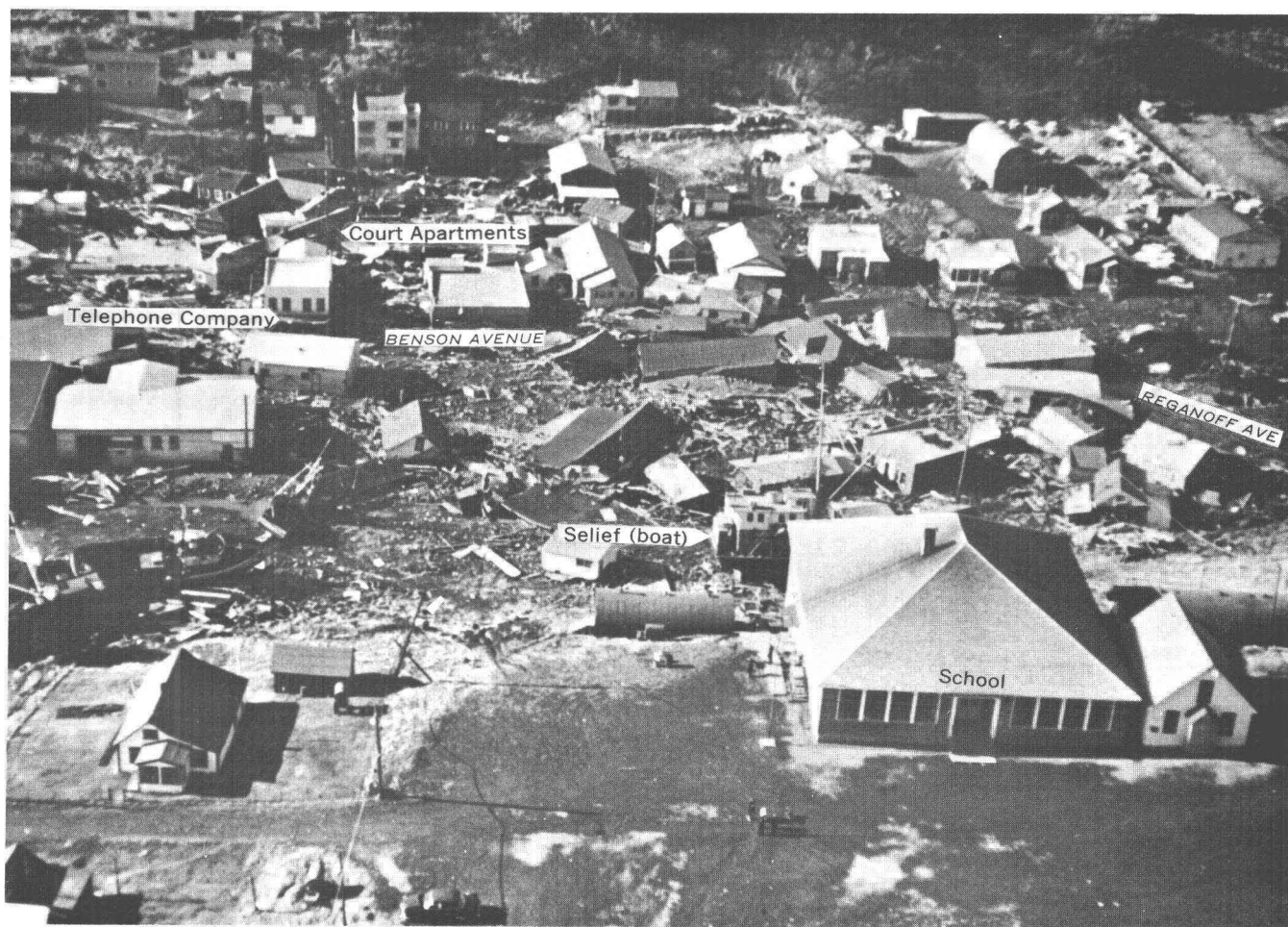
17.—Structures displaced by seismic sea waves, downtown Kodiak. View is west toward intersection of Benson and Reganoff Avenues. Photograph by Mr. Alf Madsen, Kodiak, March 1964.
