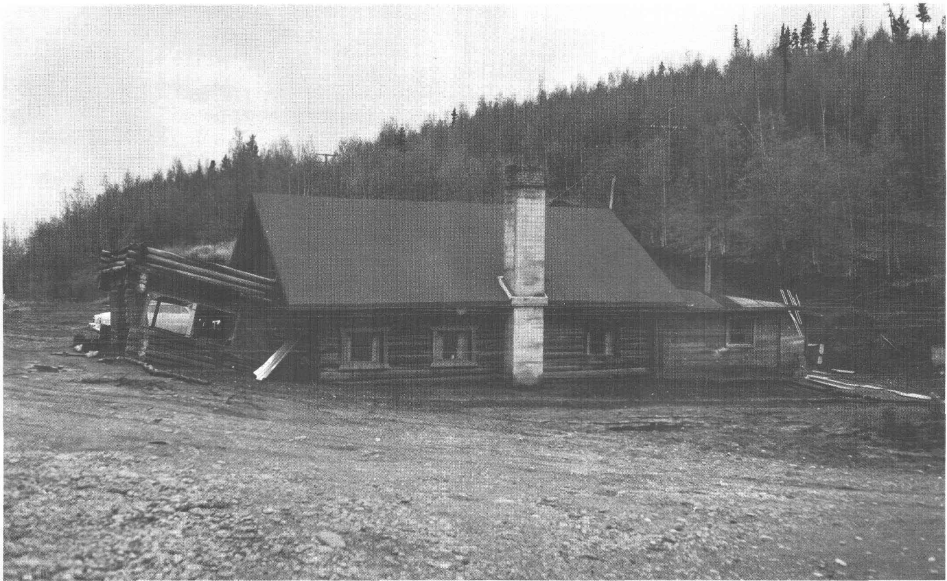
FIGURE 33.—Roadhouse, mile 278.5, Richardson Highway. The structure is distorted because of thawing of the underlying ice-rich permafrost in fine-grained silts and sands. Photograph by T. L. Péwé, May 29, 1962.
