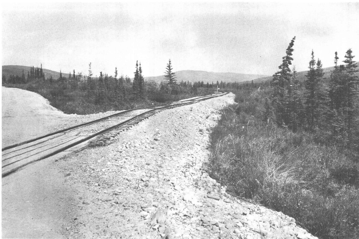
FIGURE 19.—Differential subsidence caused by thawing permafrost along the Murphy Dome Spur of the Alaska Railroad. Roadbed is in Goldstream valley and is underlain by silt. Photograph by T. L. Péwé, June 1954.
