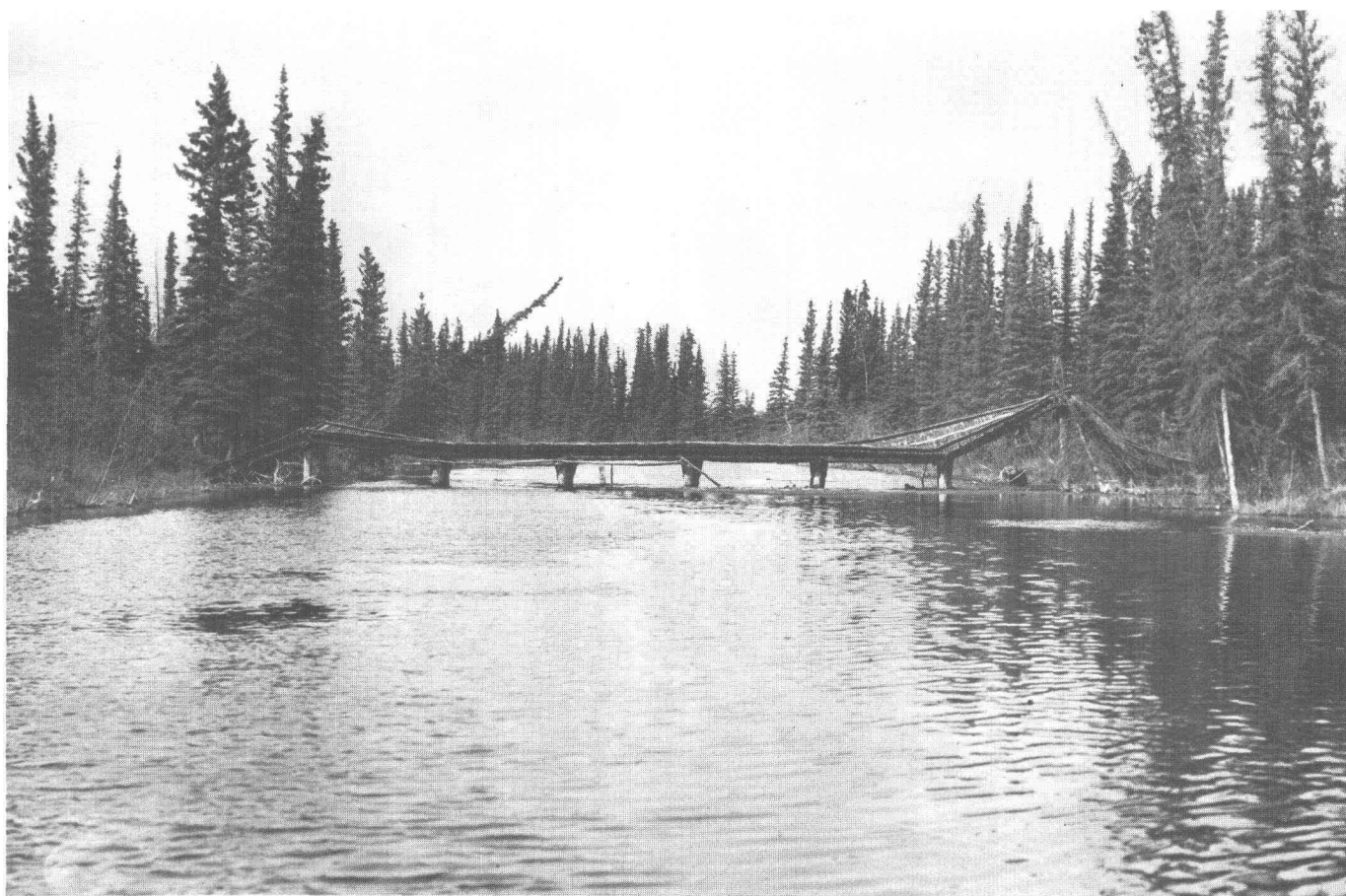
FIGURE 30.—Frost-heaved piling of bridge spanning outlet of Clearwater Lake, 8 miles southeast of Big Delta. Piles are of wood. Photograph by M. F. Meiser, August 1951.
