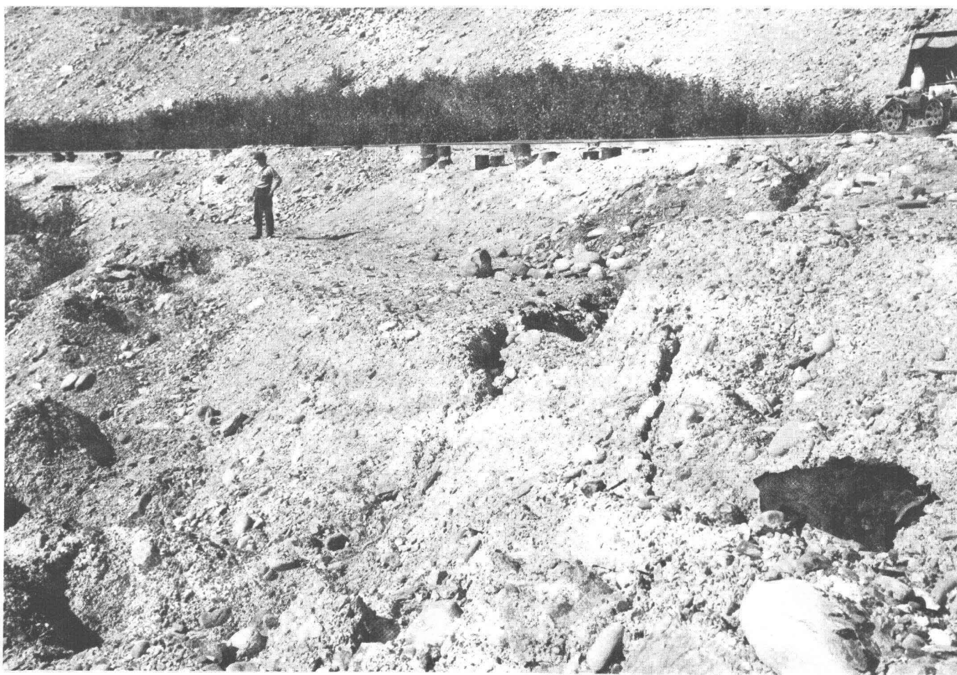
FIGURE 22.—Landslide area at mile 353.5, The Alaska Railroad. Note the tops of piles immediately downslope from the rails to prevent displacement of the tracks.
