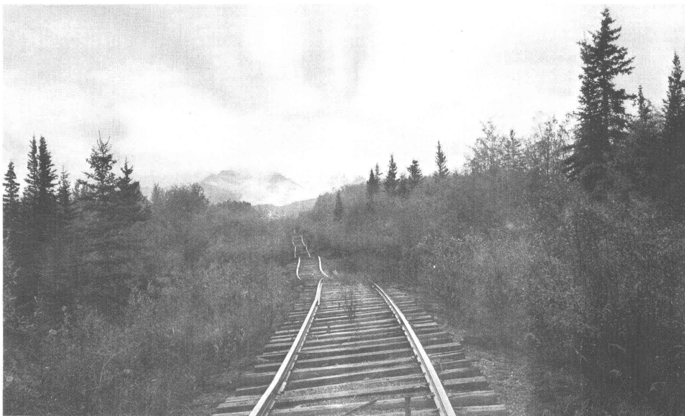
FIGURE 20.—Differential subsidence of roadbed of Copper River and Northwestern Railway near Strelna, 75 miles northeast of Valdez. The thermal equilibrium of the fine-grained sediments underlying the roadbed was disrupted during construction and the permafrost started to thaw. Maintenance and use of the railroad was discontinued in 1938. Subsidence as well as lateral displacement, however, has continued. Photograph by L. A. Yehle, September 1960.
