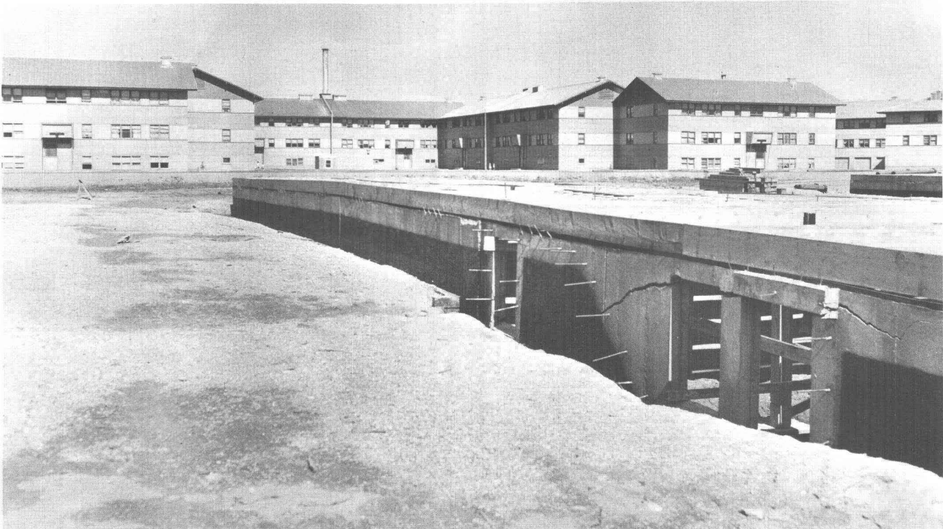
FIGURE 35.—Fracture due to frost heaving of 4-inch concrete foundation of an apartment house in Fairbanks. Photograph by T. L. Péwé, June 1954.
