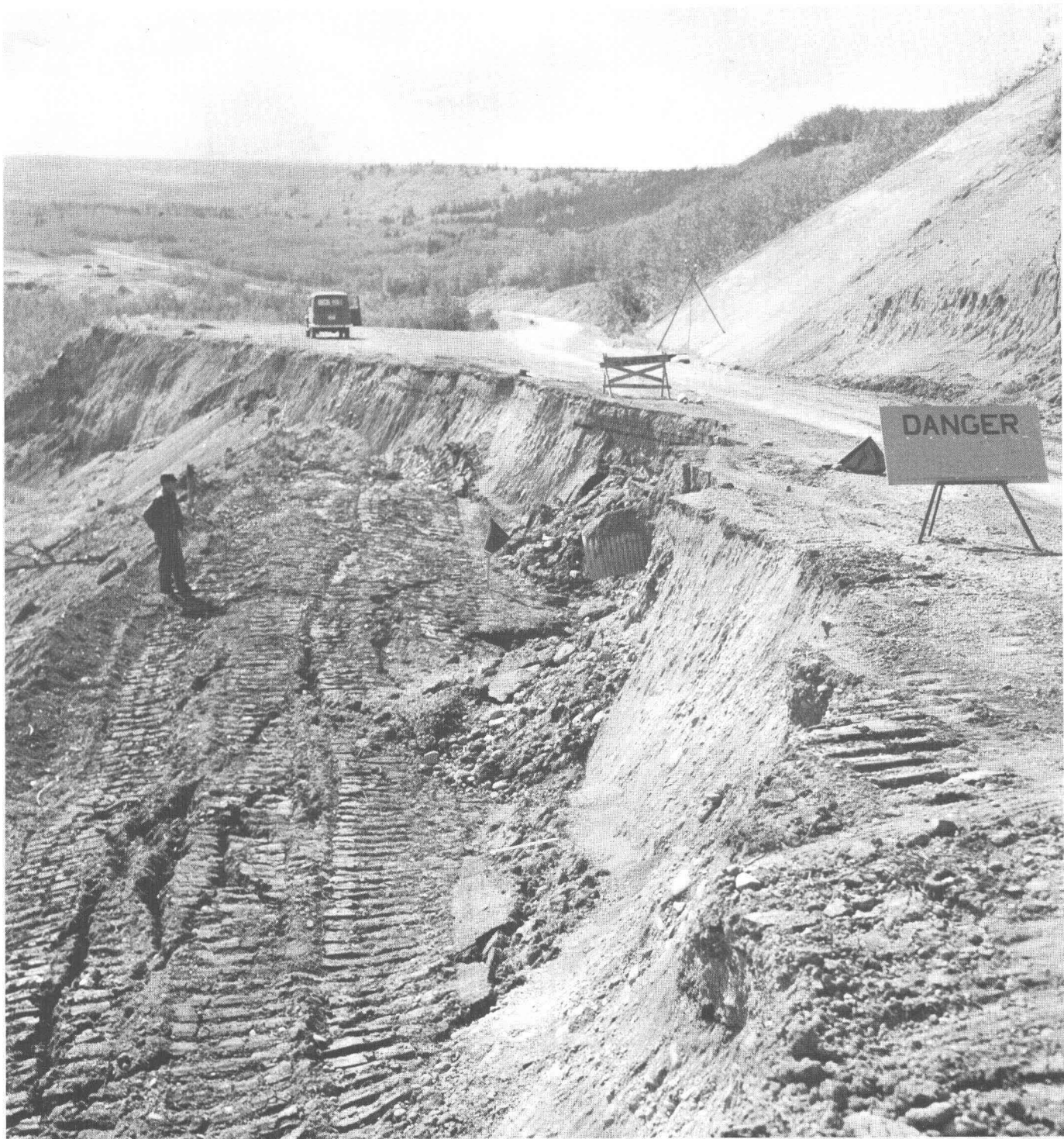
FIGURE 26.—Slump block of fine-grained highway fill material at Simpson Hill, near mile 113 on the Richardson Highway. Centerline of road formerly lay over exposed part of sheared culvert. Note bulldozer tracks on slump block surface, which are a continuation of those at road level on right side of photograph. Photograph by D. R. Nichols, September 1955.
