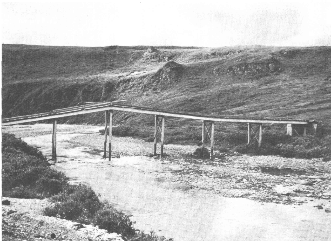
FIGURE 32.—Frost-heaved steel-pile bridge spanning North Fork at about mile 120 on the Kougarak Highway, Seward Peninsula. Photograph by G. D. Eberlein, summer 1955.
