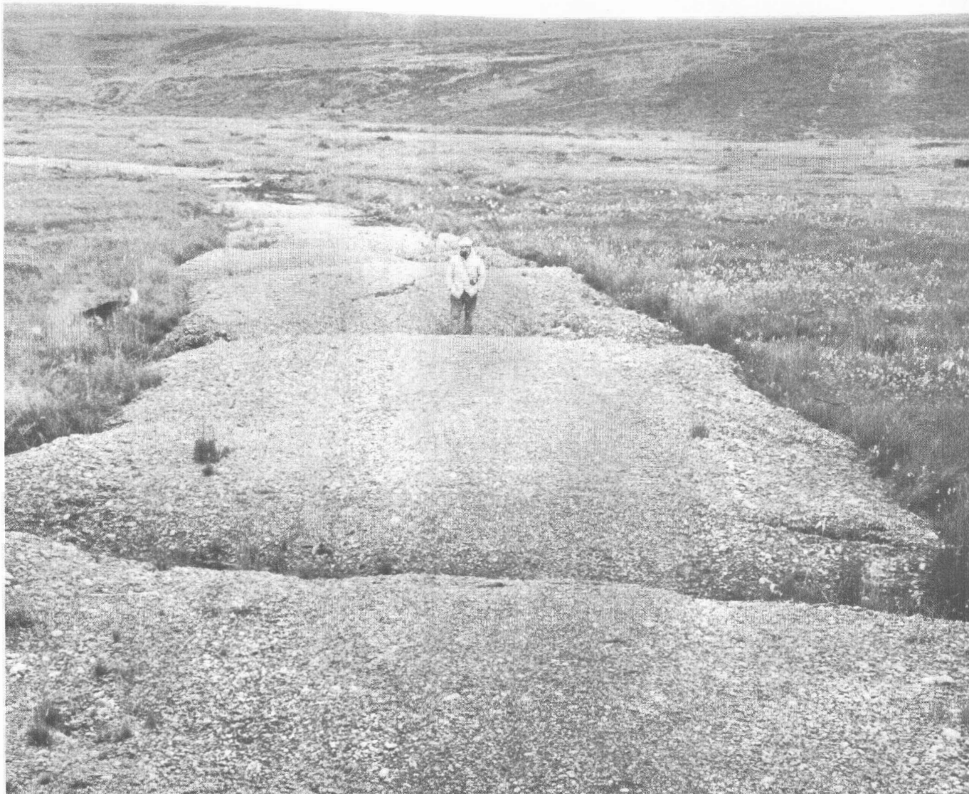
FIGURE 25.—Gravel road near the Umiat showing severe differential subsidence caused by thawing of ice-wedge polygons in permafrost. Photograph taken in August 1958.
