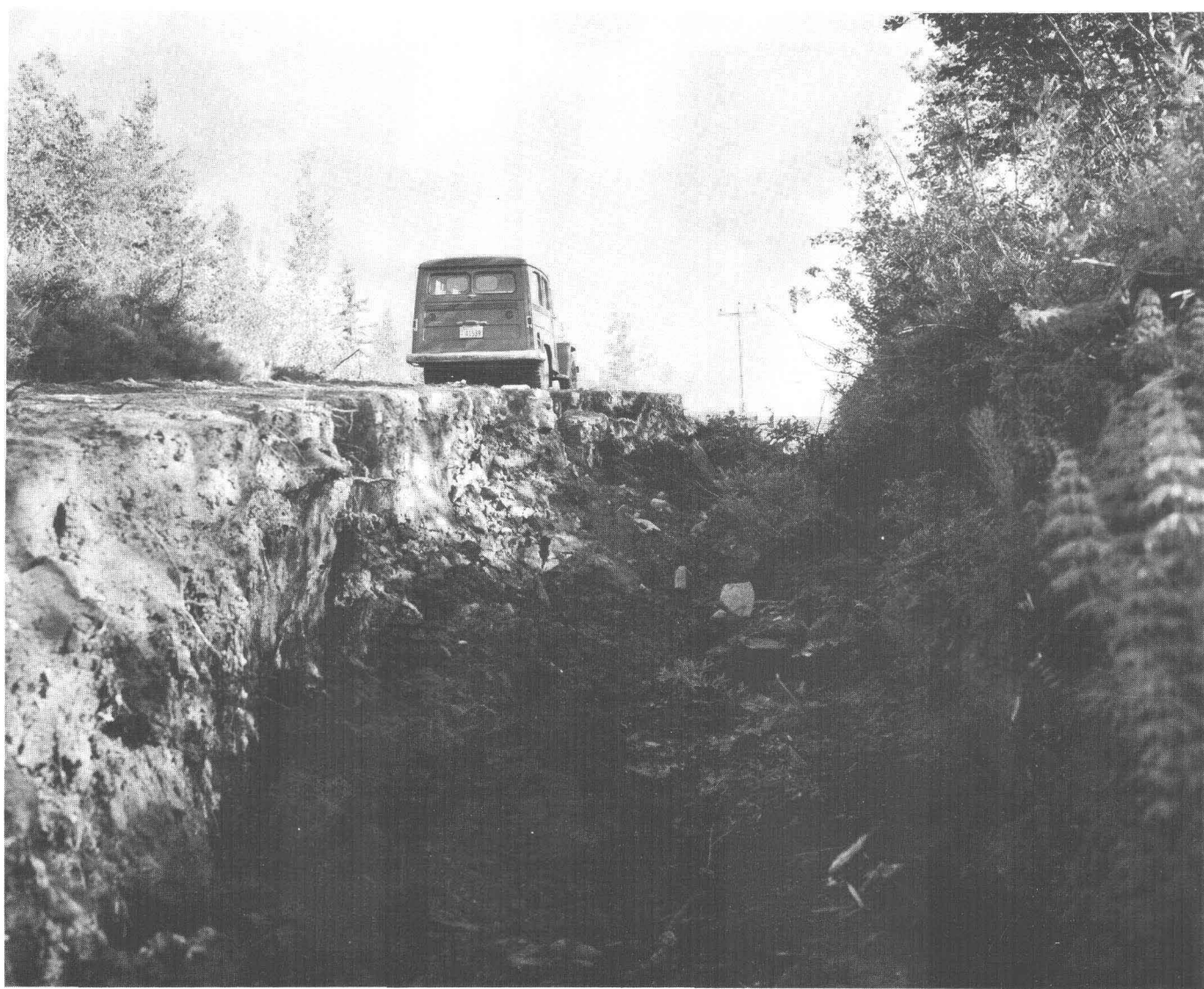
FIGURE 27.—Old Sheep Creek Road northwest of Fairbanks. Gully along edge of road was caused when the surface drainage thawed the permafrost in the underlying loess deposits. Photograph by T. L. Péwé, summer 1955.
