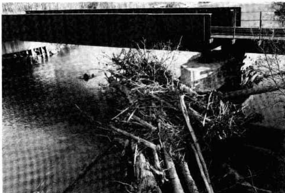
Figure 16.--Debris lodged on bridge pilings, Resurrection River.
