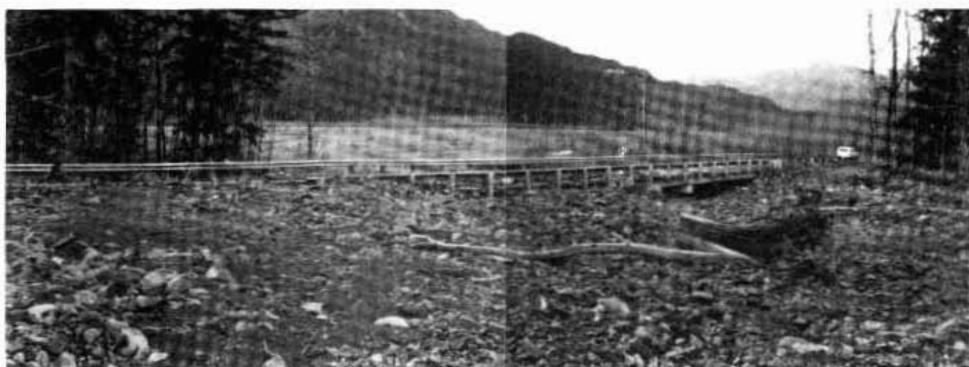
Figure 13.--Cobble and gravel deposits at Bridge 1389, mile 4.7 Exit Glacier Road. View downstream on October 13, 1986.
