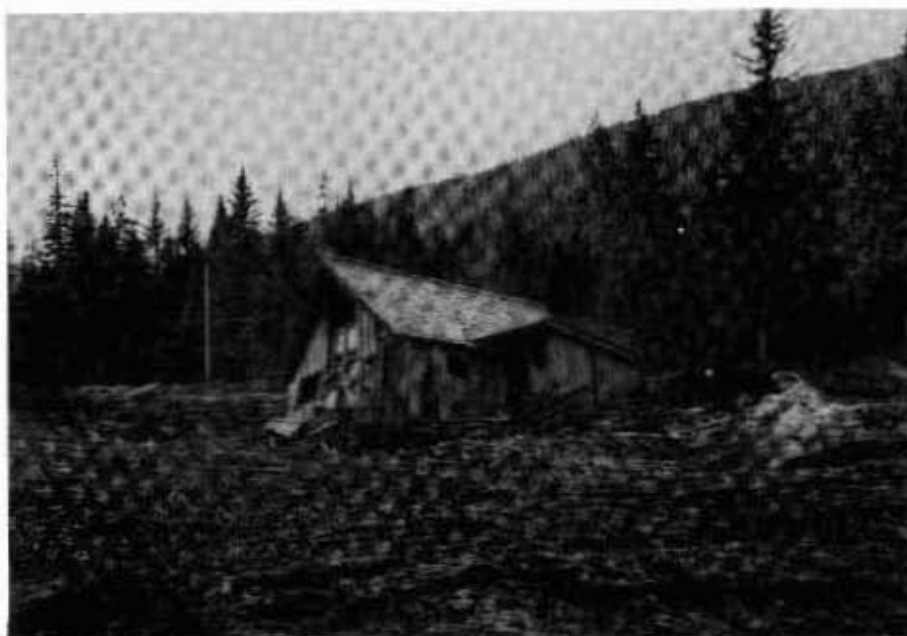
Figure 11.--Flood and debris damage to residence on the Lost Creek alluvial fan.
